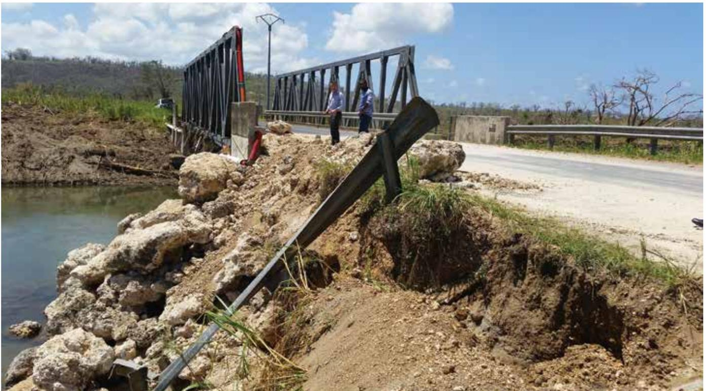
missed the northern provinces of Torba and Sanma, the associated rain caused flooding damage to culvert crossings, road pavements, and aerodromes in these two provinces.<sup>38</sup>
