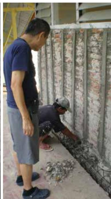
**Figure 9.** An unreinforced masonry school building (left) has its walls strengthened with chicken wire mesh (right)
