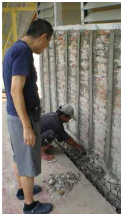
**Figure 9.** An unreinforced masonry school building (left) has its walls strengthened with chicken wire mesh (right)
