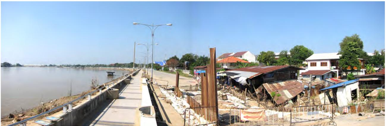
**Figure 12:** Aboveground damage from underground sewage pipe network subsidence (16 Nov 2011)
