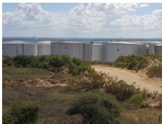
Damaged infrastructure at Nacala port
