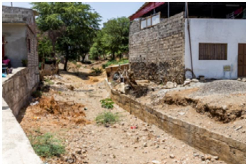
**Picture 8:** In the socially deprived neighborhood of Safende in Praia, this drainage canal appears to have more capacity upstream than downstream.
