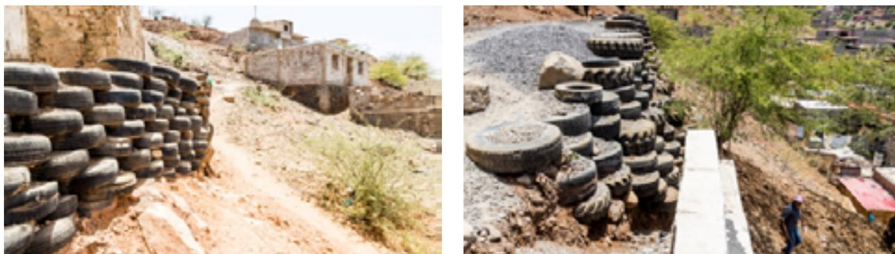
**Picture 10:** These improvised erosion mitigations might not withstand torrential rainfall. Houses below are directly at risk.
