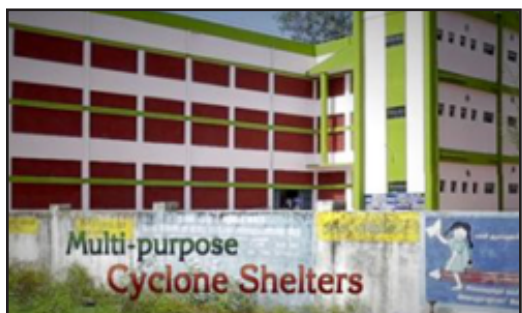
Supporting Multi-Purpose Cyclone Shelters (2016)
