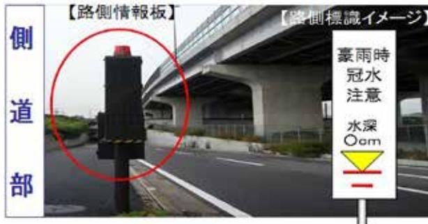
A sample notice on this roadside electrical information board, if the alarm light were on, would note in red light, "Caution! Flooded due to rain. Water depth 30 cm."
