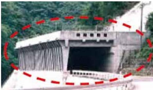
Shelters against rock, debris, and snow are often built over roadways adjacent to steep slopes. There is no substantial difference between shelters that protect against rock or soil fall and those built for snow avalanches. They usually serve both rock or soil fall and snow avalanches in a snowy region. The material of the shelter is three types: reinforced concrete, prestressed concrete, and steel.
