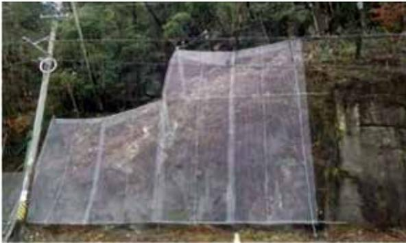
Wire netting (rockfall net) is subdivided into covering type and pocket type (shown in the photo, left). The covering type tightens loose rock mass and stops these from falling through the tensile force of the wire net. The pocket type is a barrier to protect roads against rockfalls from reaching the road, while the flexible net does not break and buffers the falling rock energy and retains the rockfalls on the mountainside of the road.
