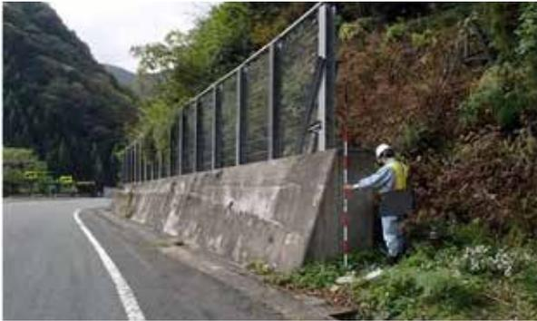
Concrete retaining walls are often used as the foundation of fences to prevent falling rocks. Energy absorption capacity of 45–650 kilojoules (kJ) was the norm; however, recently, a rockfall prevention fence capable of high energy absorption up to 1,000 kJ has been developed, and in the MLIT's New Technology Information System (NETIS).
