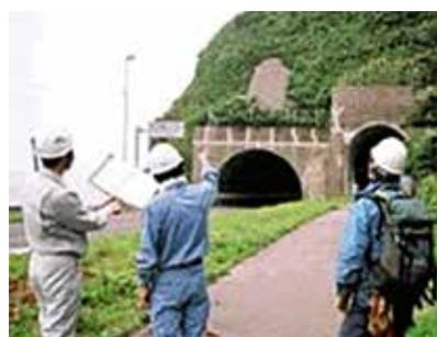
Distant-view observation is needed for proper understanding of the entire slope.
