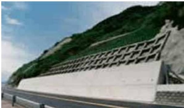
Slope stabilization measures here use a retaining wall, a slope framework (grid beam) with anchoring, shotcrete, and vegetation (bioengineering).
