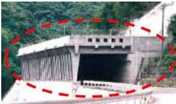
Shelters against rock, debris, and snow are often built over roadways adjacent to steep slopes. There is no substantial difference between shelters that protect against rock or soil fall and those built for snow avalanches. They usually serve both rock or soil fall and snow avalanches in a snowy region. The material of the shelter is three types: reinforced concrete, prestressed concrete, and steel.
