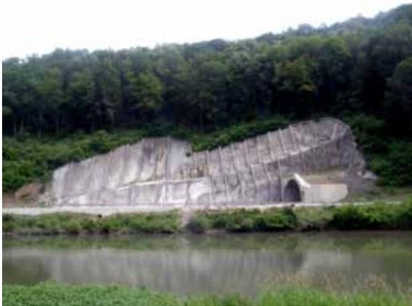
**Photo 5.5 Use of Anchors, Wire Nets, and Geotextile as Reactive Measures on Cuts, Corridor X, E-80 (LOT1-Prosek-Tunnel Bancarevo)**
