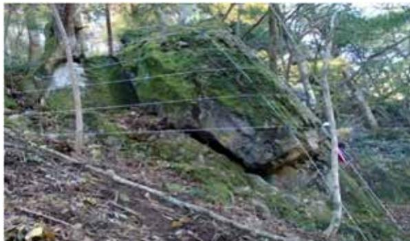
Unstable rock mass is stabilized here using steel wire rope with anchoring to prevent collapse.
