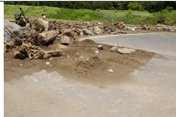
Figure 5: Damage to the runway surface at the end of runway 60.
