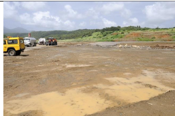
Figure 4: A large part of the apron has been washed away.
