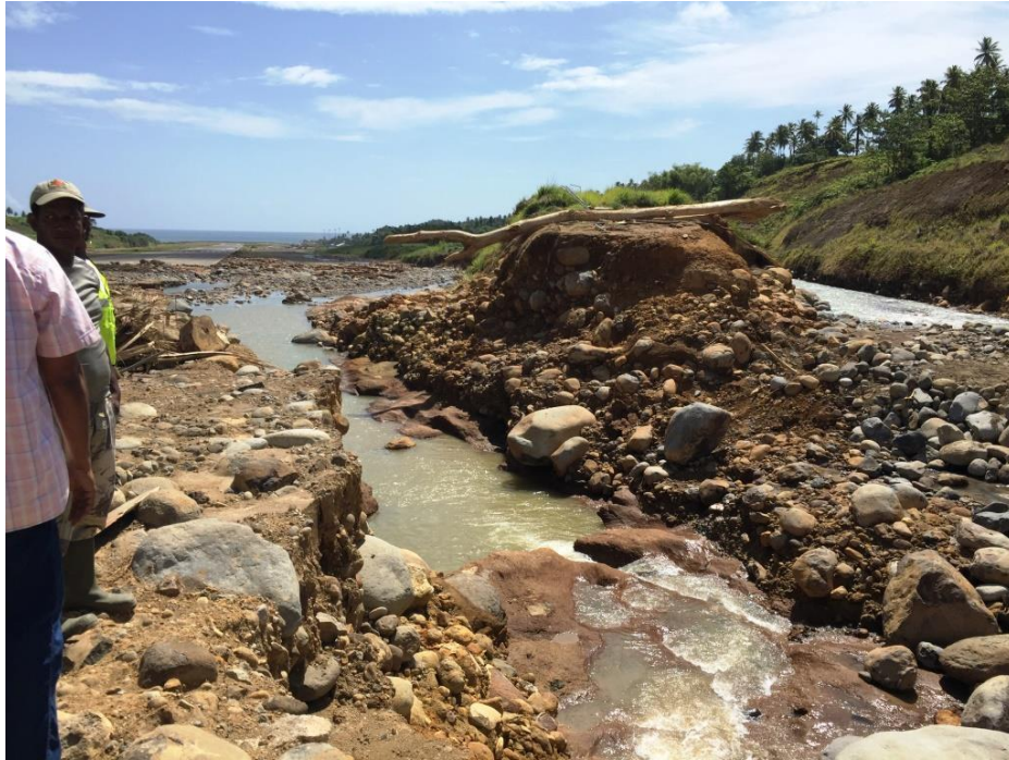
Collapse of Barrage which Caused Inundation of the Airport
