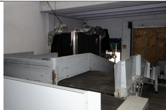
Figure 3: All luggage handling equipment, such as this x-ray machine and luggage conveyer, were rendered inoperable.
