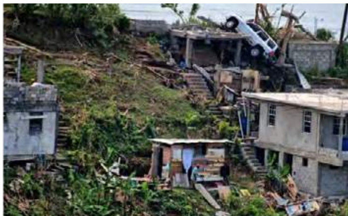
Destruction following TC Maria in Dominica in September 2017. Source: World Bank
