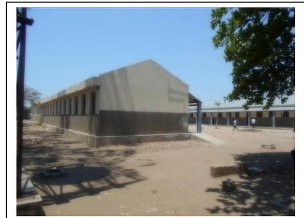
Observation: Concrete rain gutter erected to protect the bottom of roof sheet
