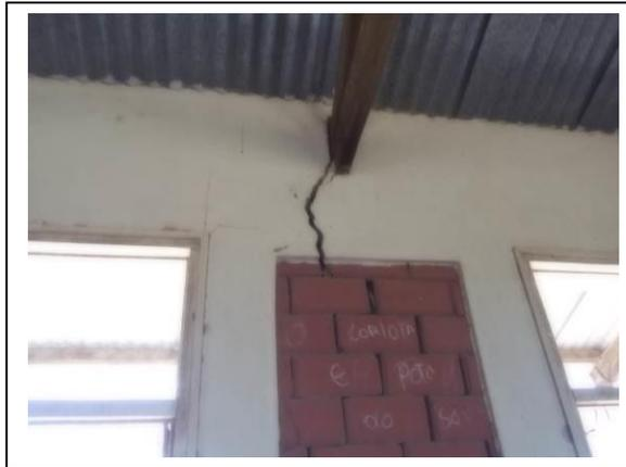
Observation: Cracks i wall/truss support
