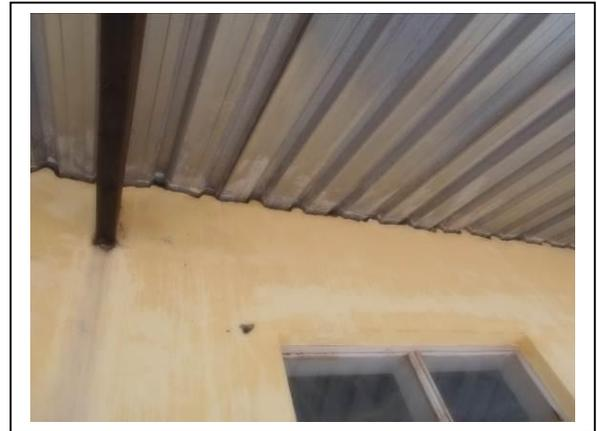
Observation: cracking between the wall and roof sheet due the effect of wind
