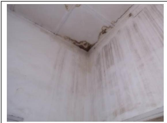
Observation: water leaking on ceiling.
