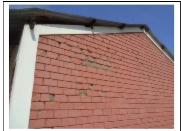
Observation: Blocks in an advanced state of degradation
