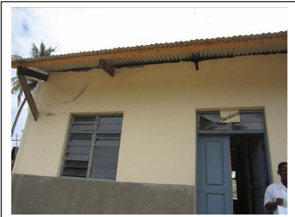
Observation: Cracking between wall and roof structure
