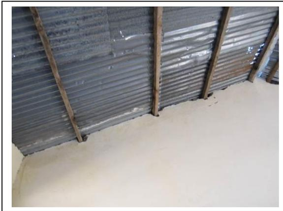
Observation: Cracking between the wall and roof
