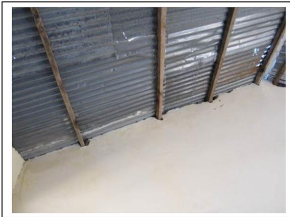
Observation: Cracking between the wall and roof
