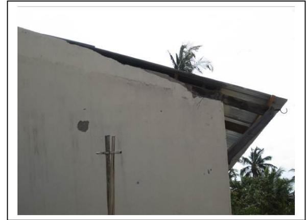
Observation: Cracks between wall and roof
