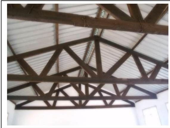
Observation: Reinforced roof structure to support the action of wind
