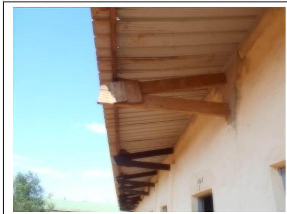
Observation: Poor repair of the roof structure
