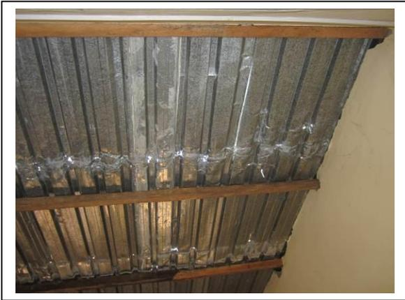
Observation: Detail of damaged roof sheet
