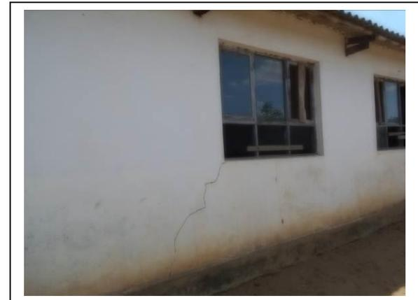
Observation: cracks are supposed to be caused by an earthquake in the old building
