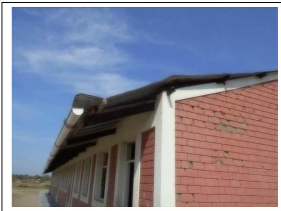
Observation: Part of the roof damaged by cyclone
