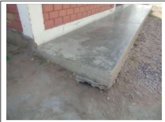
Observation: Erosion in the foundations of the walk around the building
