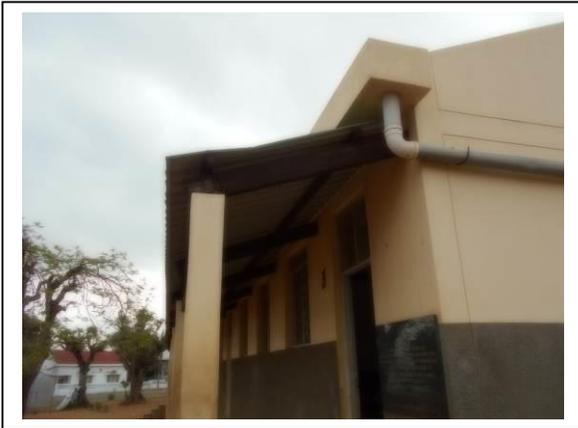
Observation: Detail of gutter constructed to collect rainwater and also to protect the roof sheet from winds
