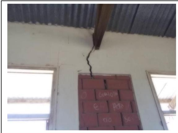
Observation: Cracks i wall/truss support
