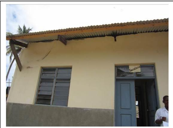
Observation: Cracking between wall and roof structure
