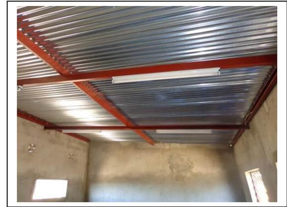
Obser: roof steel structure to upgrade (no enough slope)
