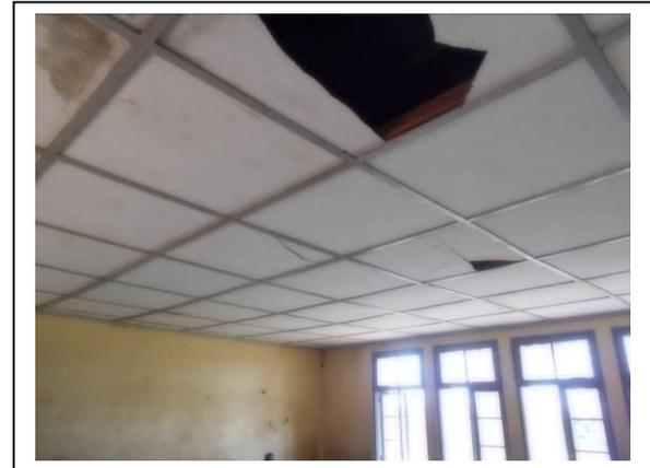
Observation: Ceiling in advanced state of degradation
