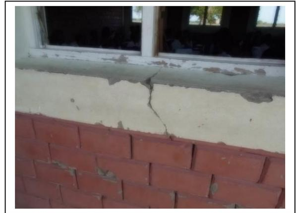
Observation: Crack at the edge of the window
