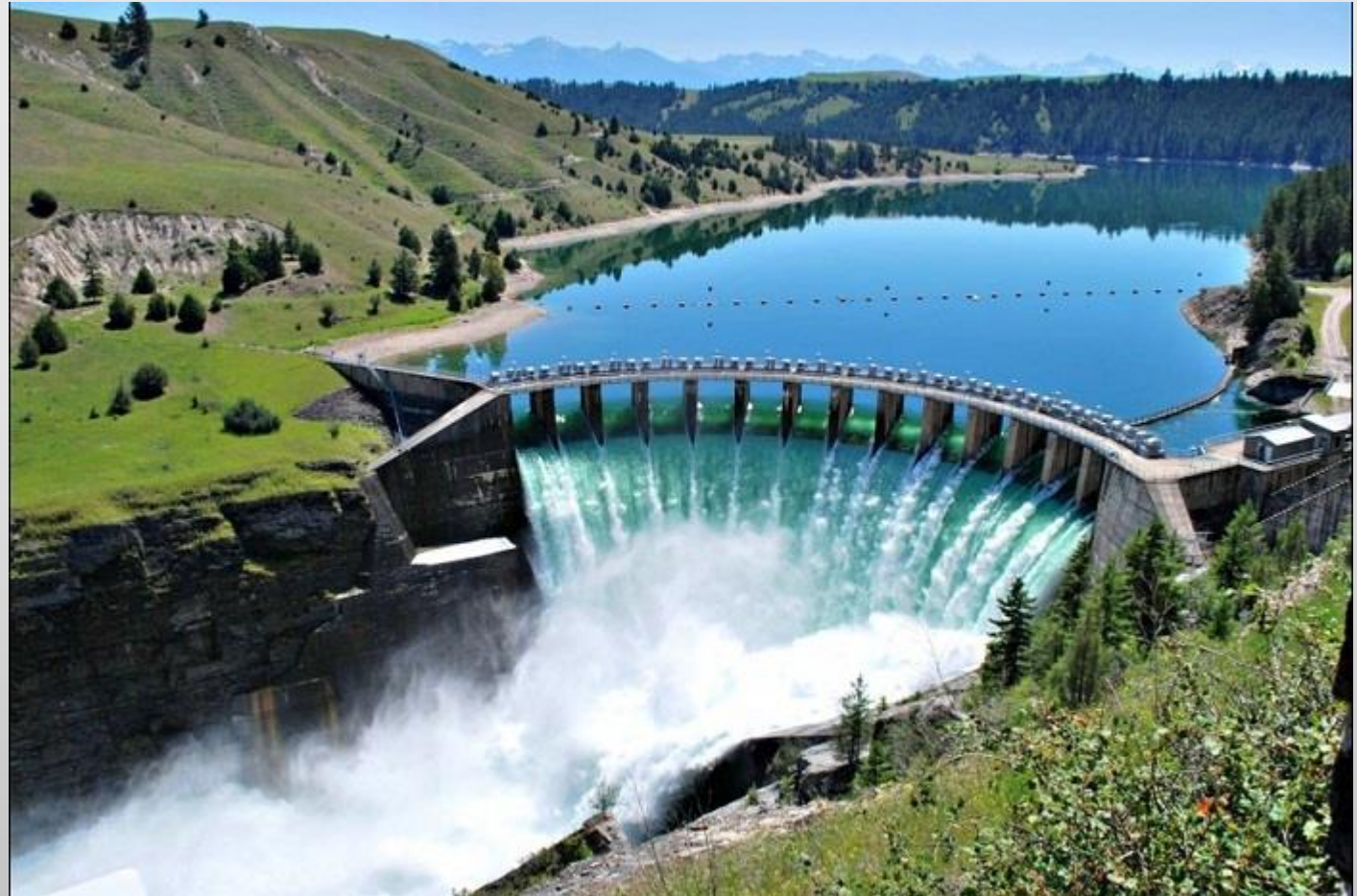
Construction Review Online/ Laúca Hydropower plant, Angola
