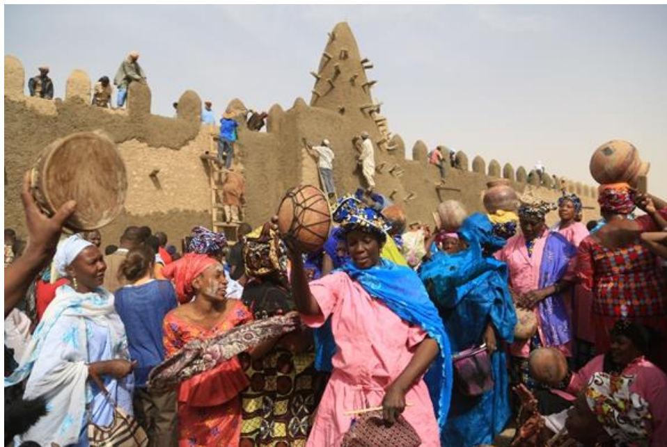
Plastering Mosque Djingareyber in Timbuktu, Mali, February 2017 © UNESCO / Modibo Bagayoko
