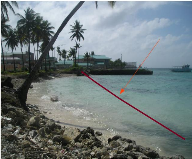
Figure 12: The red line shows the seawall that has been washed away over the years. This area has an inundation of approximately 6 meters over the period of 5 years .
