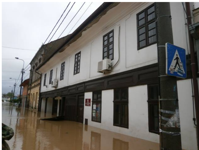
Figure 1-37. Flood Damages in Obrenovac:
