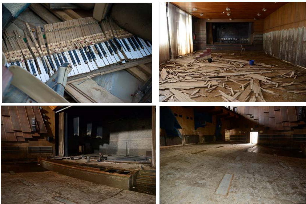
Figure 1-38. Cultural centre of Obrenovac. The situation after the withdrawal of water. The picture top right shows the small theater hall, the line of flooded level is evident. The two pictures bottom right and left show the great theater hall after the remove of barterre seats and the damages to the revolving rotation svstem of the theatre stage. from ordinary activities (restaurant, cinema tickets, renting rooms, as well as extra activities as events and sport activities) is lost for all the time of closure. The local city summer festival, planned every year, will probably not take place. The calculation takes 79 salaries at risk x 6 months: 266,400; no income from summer festival: EUR 3,000; no income from ordinary activities: EUR 210,000. Total: EUR 479,400.
