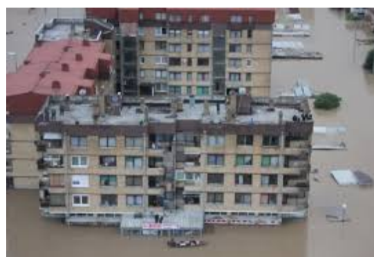
Figure 1-34. Flooded apartment blocks
