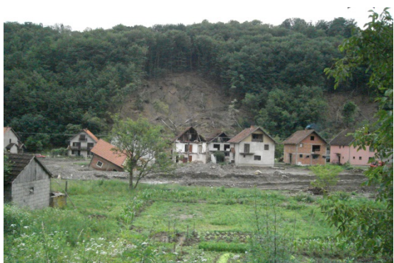
Figure 1-33. Krupanj, effects of landslides and flooding
