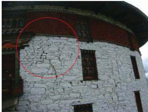
Below: Vertical Crack on the wall
