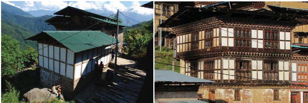
Figures above: Houses with *Eckra* type of construction
