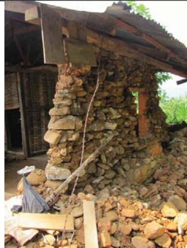
Wall cracks are a result of the stresses within the wall. Where the joints of the wall are not staggered properly, the masonry tends to open up. Diagonal opening cracks occur when the lintel band above the opening is absent. As a result, due to shear stress at the opening, these cracks may appear.
