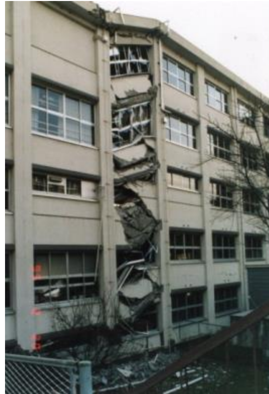
Severe damage to columns and beams
