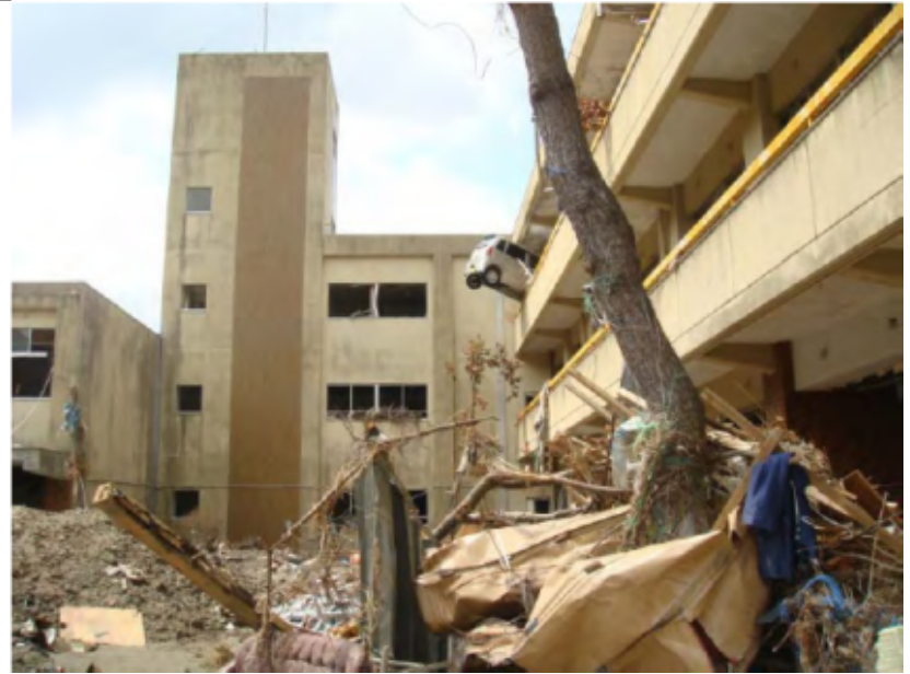
Tsunami engulfed up to the 3 rd floor of the school building
