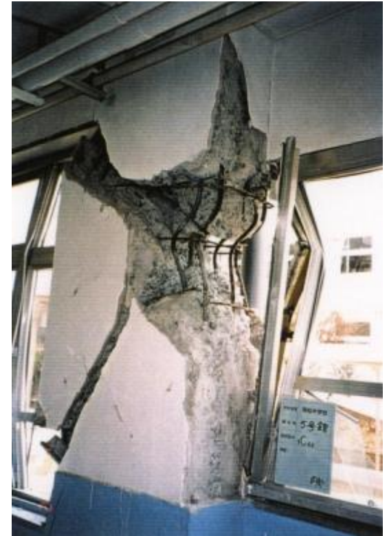
Severe damage to column
