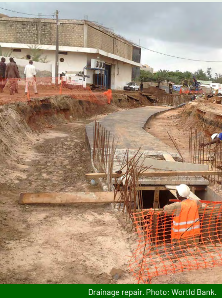
Drainage repair. Photo: World Bank.
