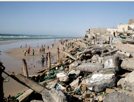
Coastal erosion in Saint Louis. Photo: World Bank.
