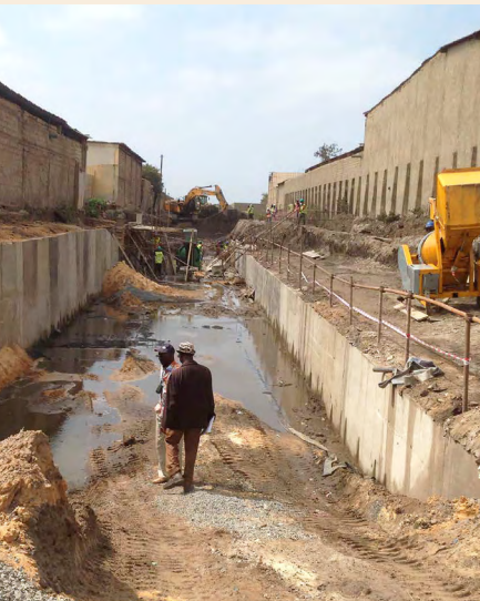
Drainage maintenance/repair. Photo: World Bank.
