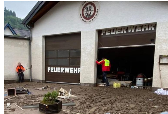
Germany, 2021 flooding of fire station Dernau
