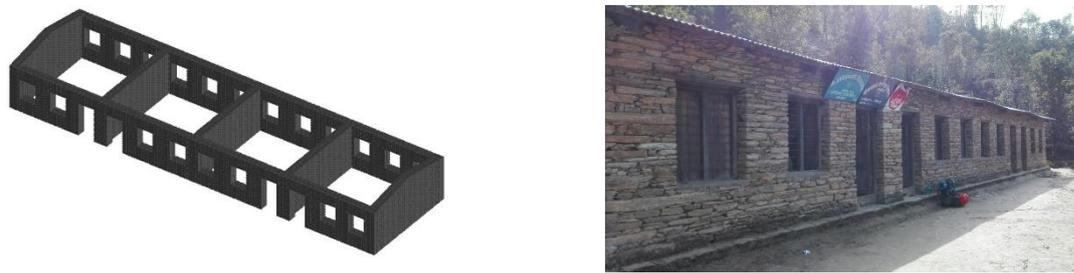
Figure 6. Dry stone masonry (UCM-URM1 Low-rise with low seismic design)-GLOSI
