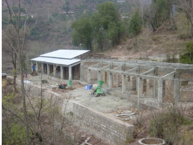
Figure 12a. SCHOOL RECONSTRUCTION IN PAKISTAN. Access to appropriate technical expertise ensured that inadequate seismic detailing was identified and amended during design review.
