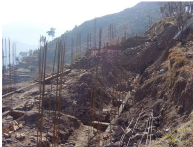
Figure 10b. SCHOOL RECONSTRUCTION, PAKISTAN. Although the school building was designed to reduce vulnerability to earthquakes the risk was still high due to the exposure of the site. Therefore major earthworks were required to protect the school from potential landslides.
