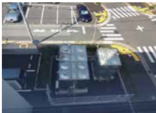
Installation of large water-collecting tank
