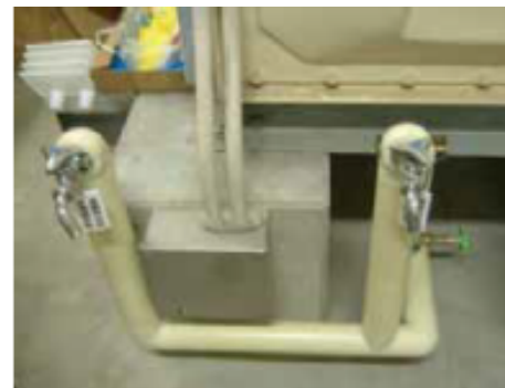
Installation of faucets to an water receiving tank
