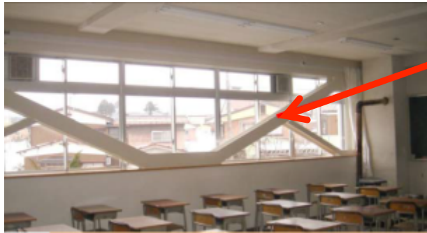
Steel brace has been added
