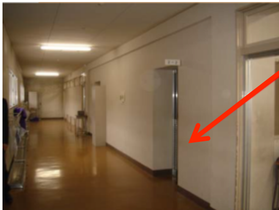
Shear wall has been added
