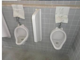
Clogged and smelly toilets due to aging
