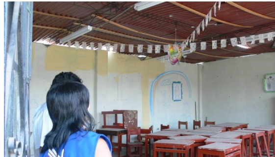
Unconfined masonry (ASC)
