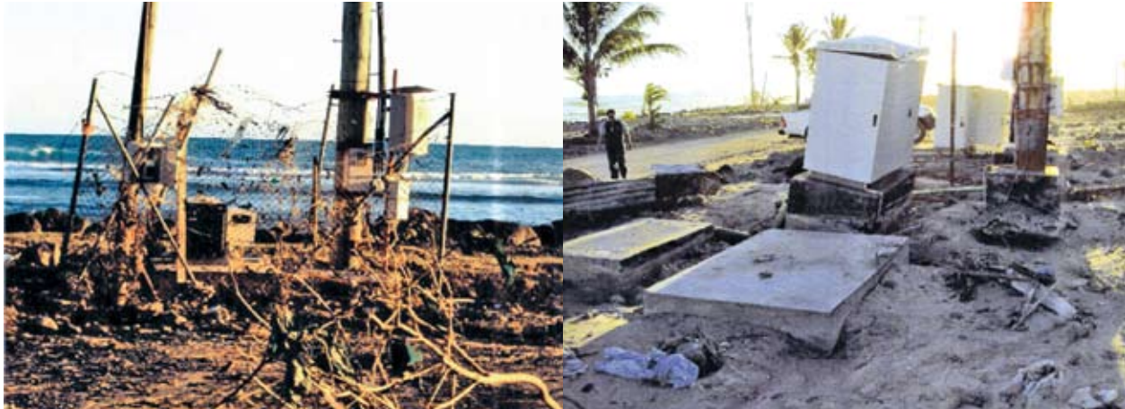
Figure 15. Damaged telecommunications sites
