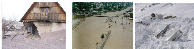
Figure 1.1: Mudflow, Flood and Avalanche related Damages in Kyrgyz Republic
