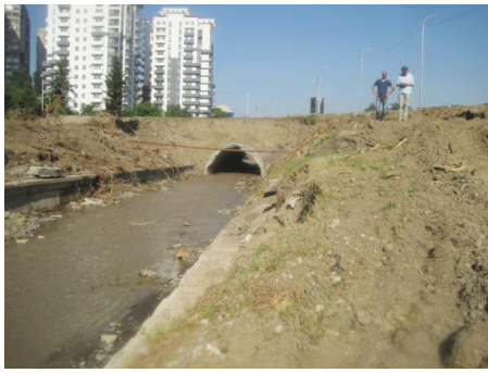
Photo 3.11 Open Vere River Channel Section after Tunnel 4
