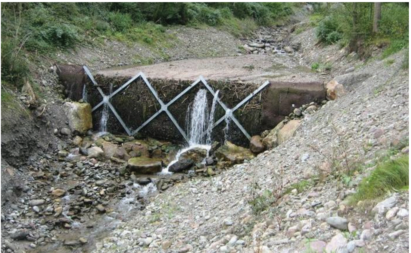
Photo E. 22. Erdox Structure for secondary watercourses
