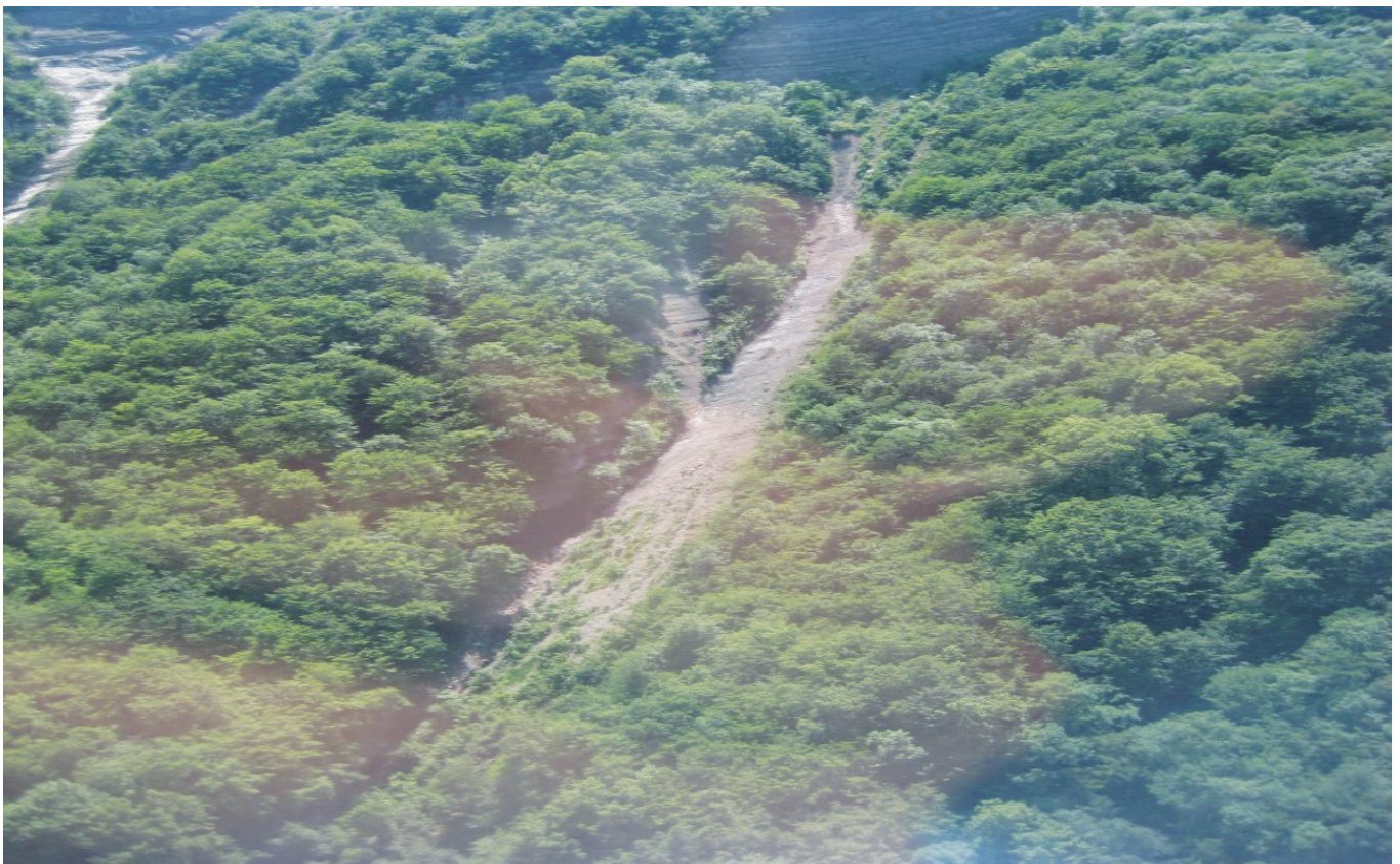
Photo E. 9. Soil Slips
