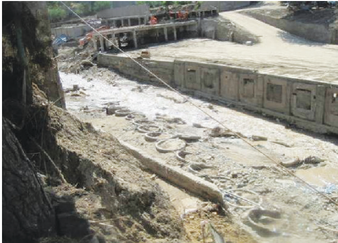
Photo 3.1 Unapproved Bridges Upstream from the 1958 Tunnel
