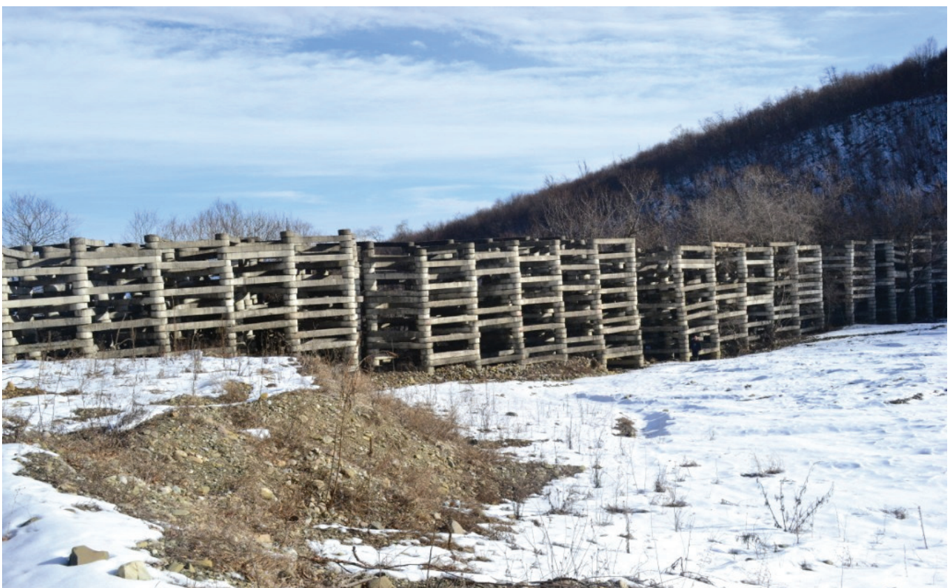
Photo E. 28. Selective Barrier to capture the floating (debris timber) transportation (Utilized in Georgia)
