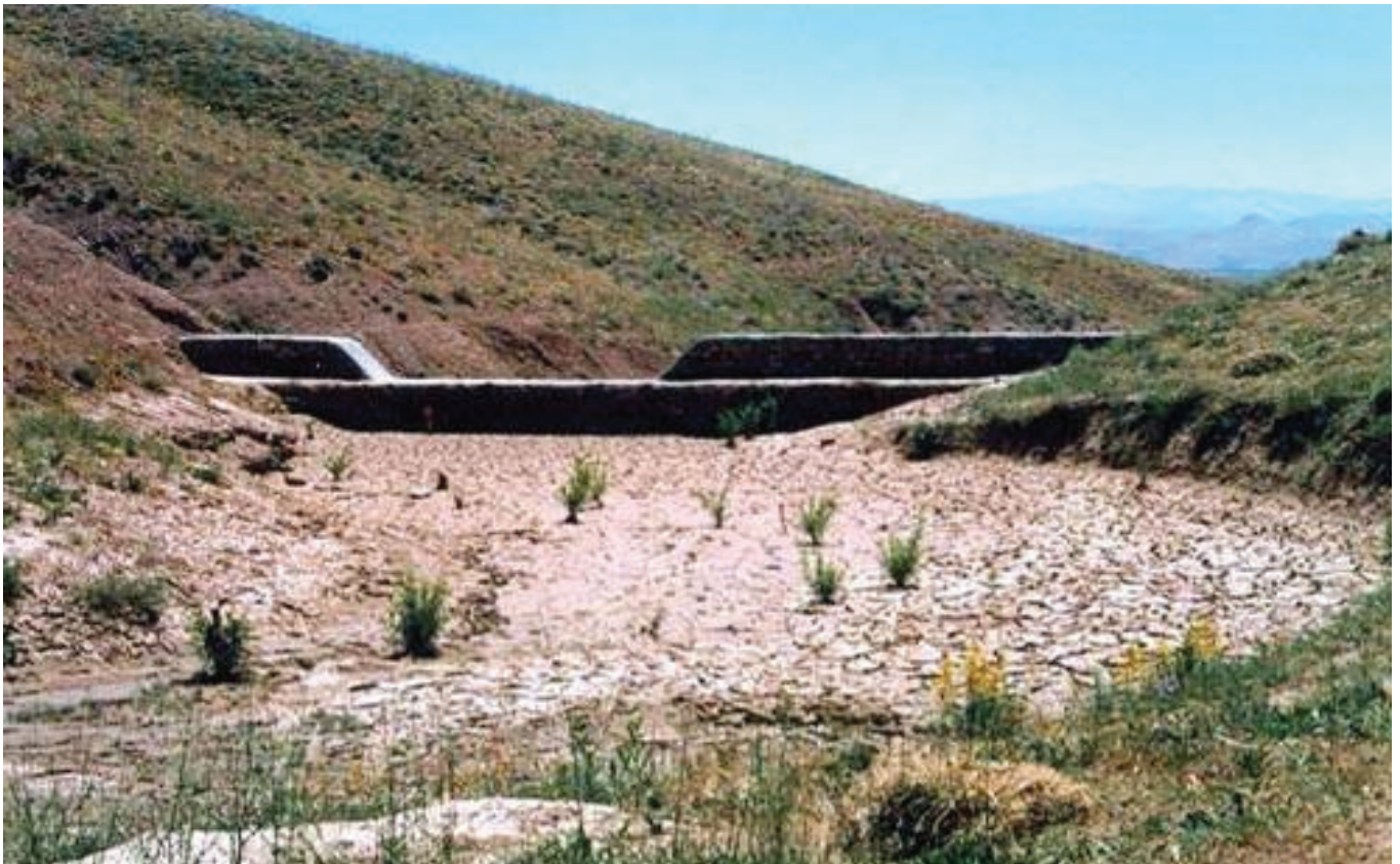
Photo E. 17. Check dam, Gabion Weir
