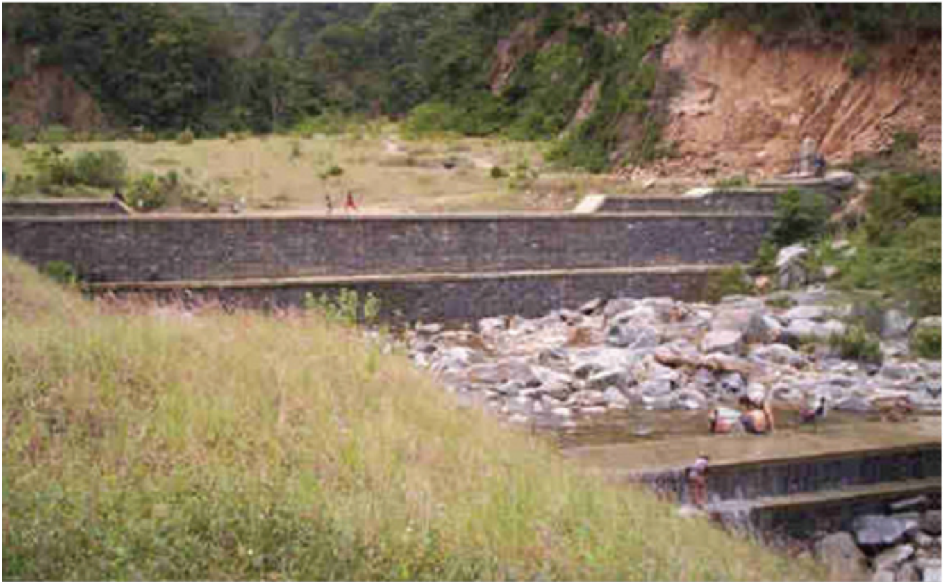
Photo E. 21. Check/selective dam, Gabion Weir
