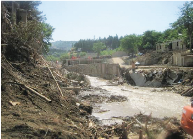
Photo D.1 River Encroachment
