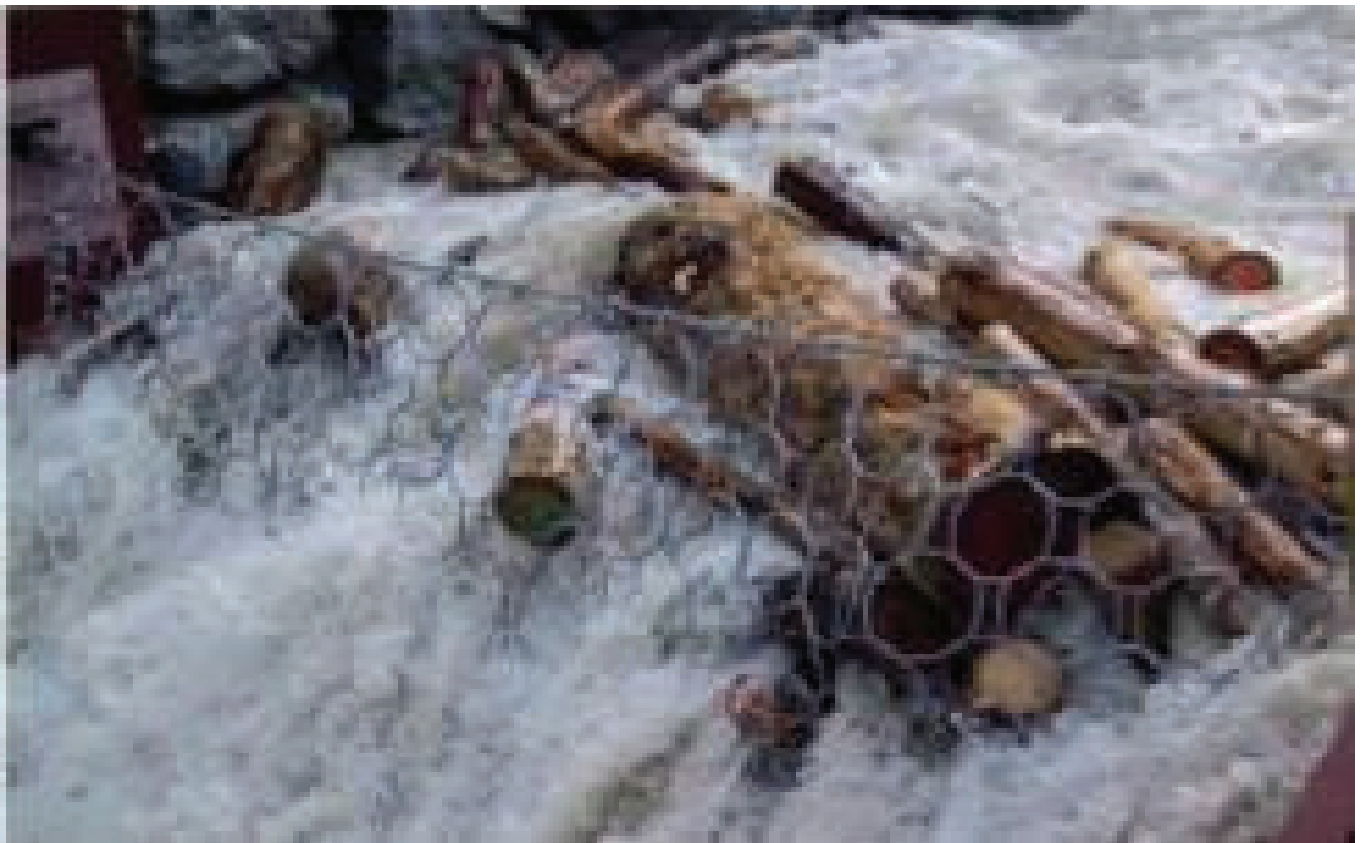
Photo E. 26. Floating Debris flow barrier for secondary watercourses,
