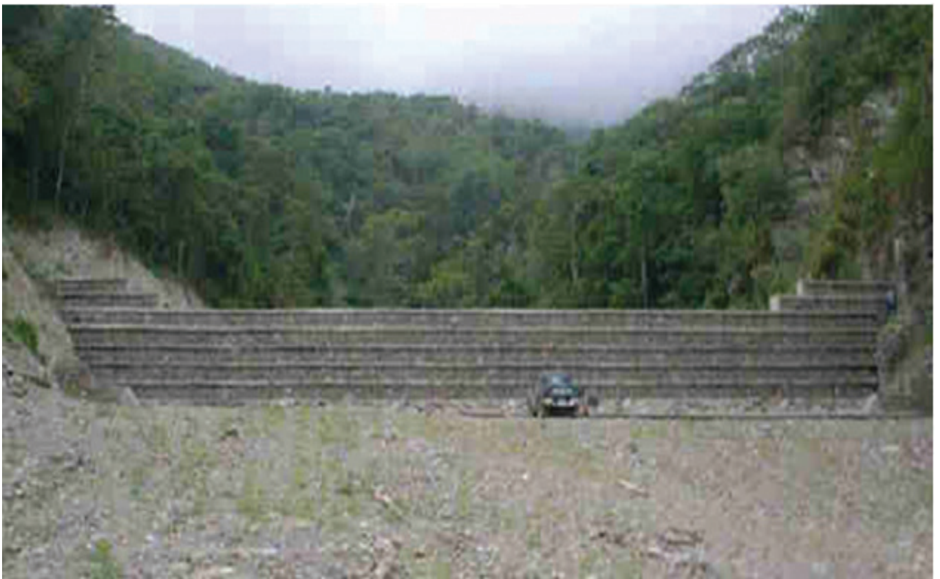
Photo E. 18. Check dam, Gabion Weir
