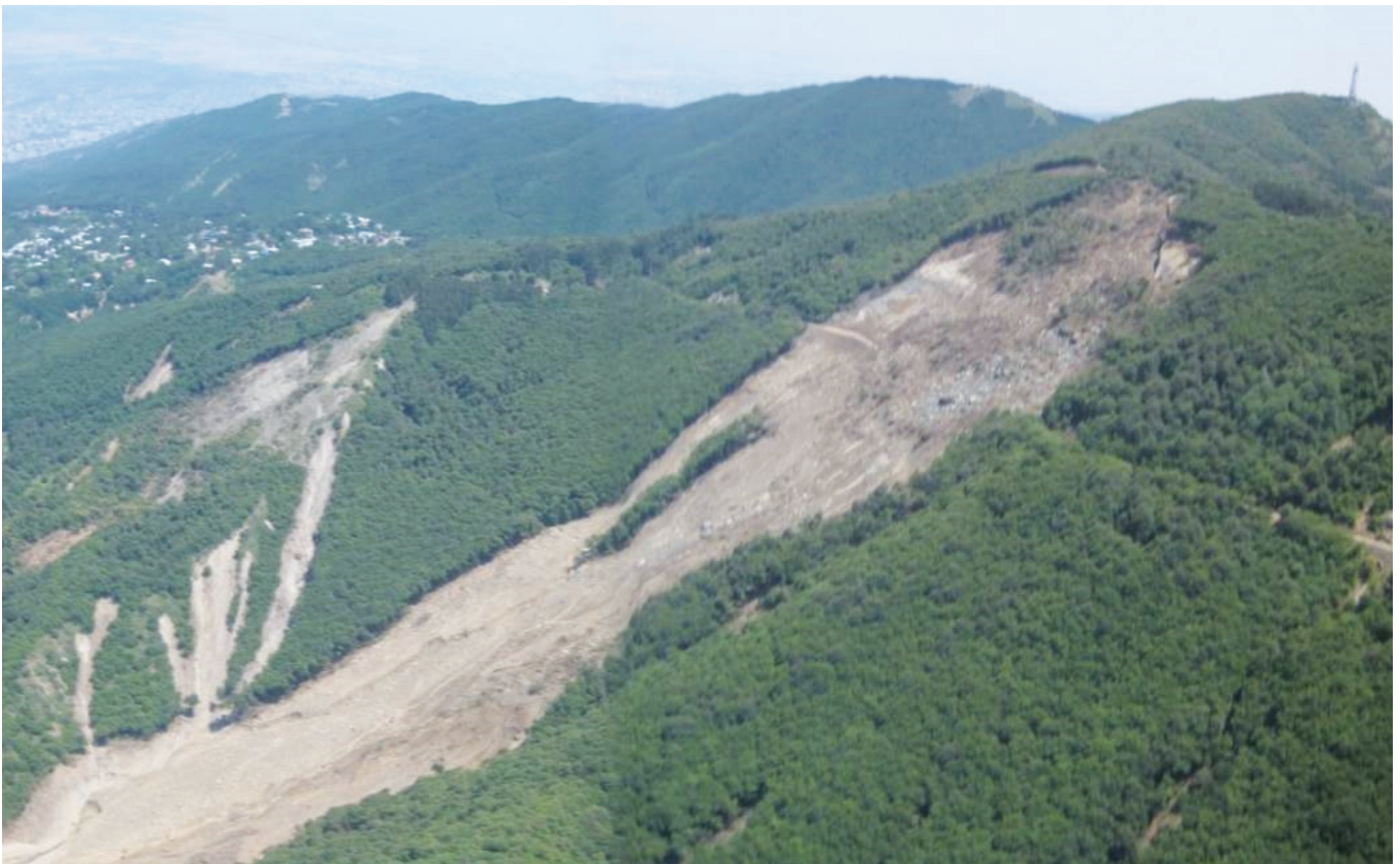
Photo E. 3. Largest landslide settled towards Akhaldaba village.
