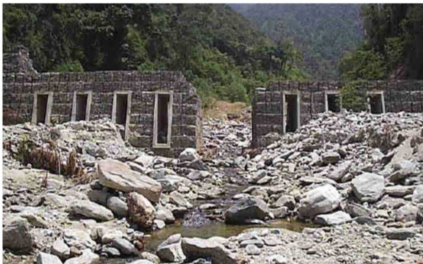
Photo E. 20. Check/selective dam, Gabion Weir
