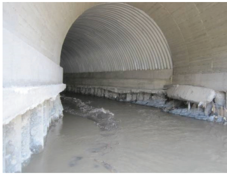
Photo 3.6 Exposed Pile caps & piles at Outlet from Tunnel 6
