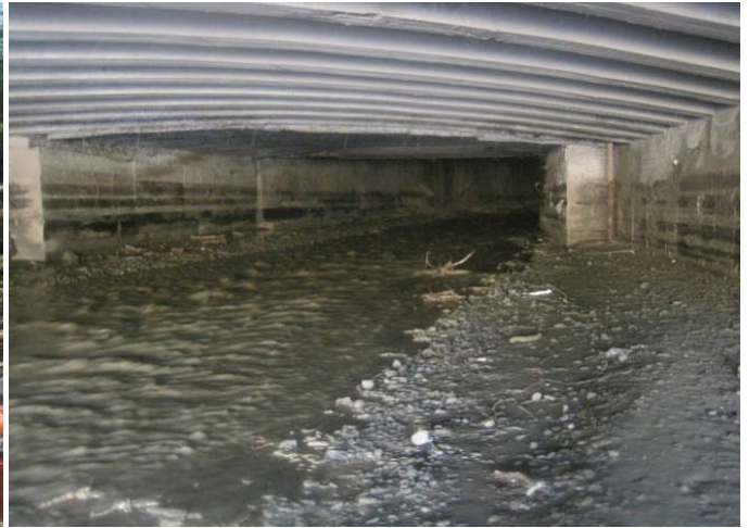
Photo D.2 Exit from Tunnel 1 at Kura River
