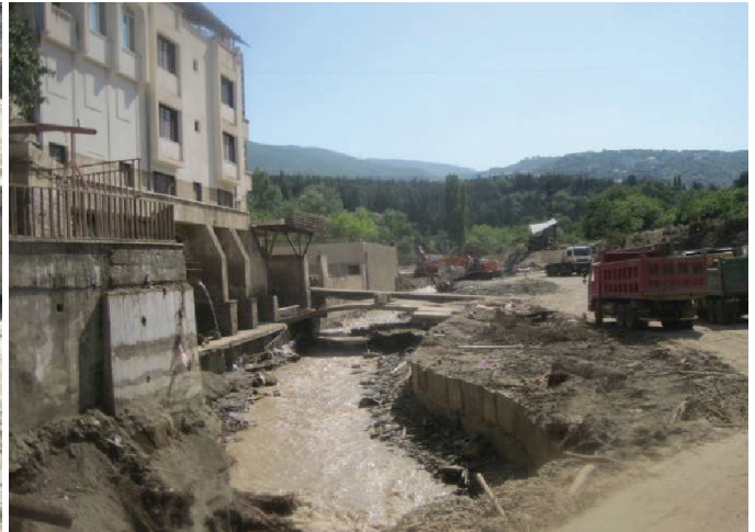
Photo 3.2 River Encroachment u/s from 1958 Tunnel
