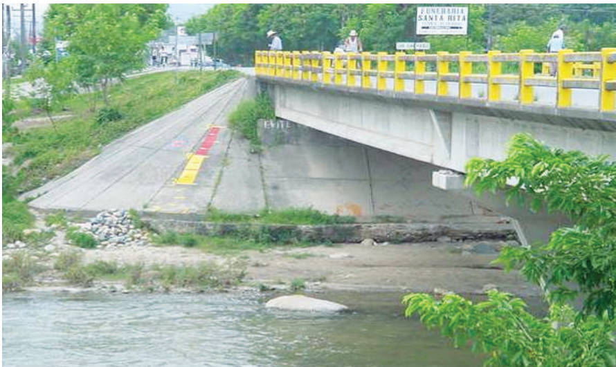
Photo E. 15. Direct control of the water level flow
