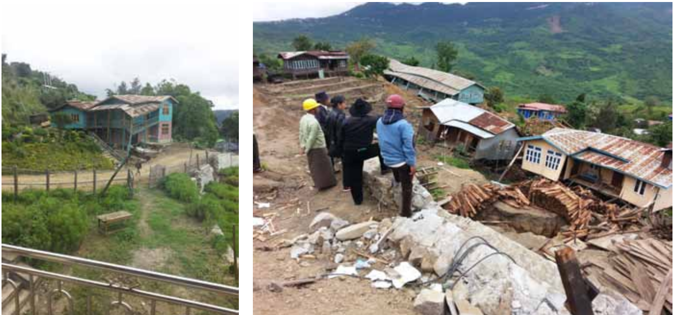
Figure 30. Damaged houses in the Chin State
