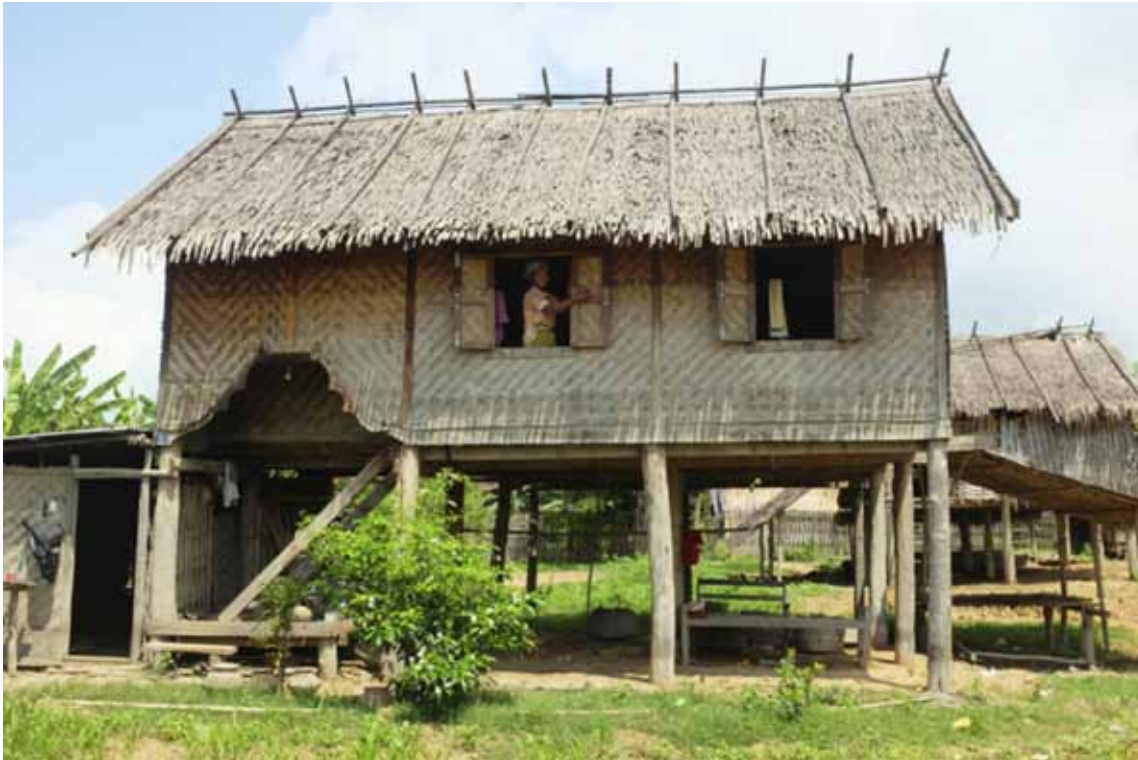
Figure 31. Damaged houses in Magway Region – mudlines (red arrows) indicate peak flood level
