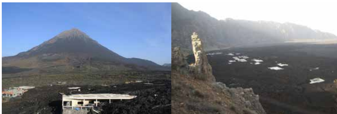
Figure 1.4: Damage to Private Properties in Portela (left) and Bangaeira (right)
