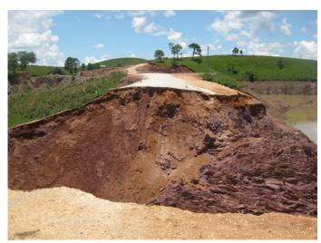
Figure 13: A section of road that was washed away in Xiengkhouang
