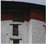
The Joint Assessment team visited the Paro *Tadzong* on 6 Oct 2011 as part of the field visit. Paro *Tadzong* has suffered major damage on some parts of its structure from the 2011 earthquake.
