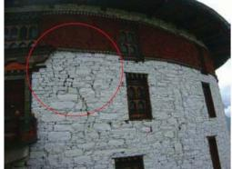
Below: Vertical Crack on the wall
