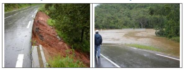
Figure 52: National Road RN 45: Flooded road and bridge and Breach
