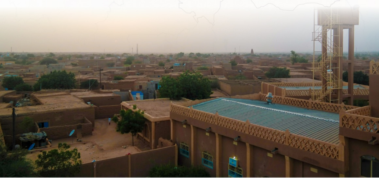
Relatively uniform building stock in the Nigerian city of Agadez.
