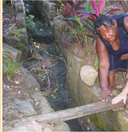
FIGURE 9.3 Maximum observed flow level in a MoSSaiC drain during Hurricane Tomas
