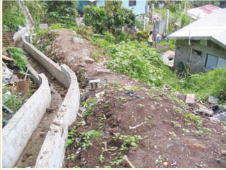
FIGURE 6.21 Drain construction above a failed slope
