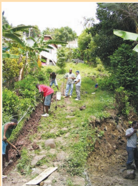
FIGURE 7.2 Contractor site meeting
