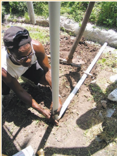
FIGURE 7.24 Household roof water connections to main drains
