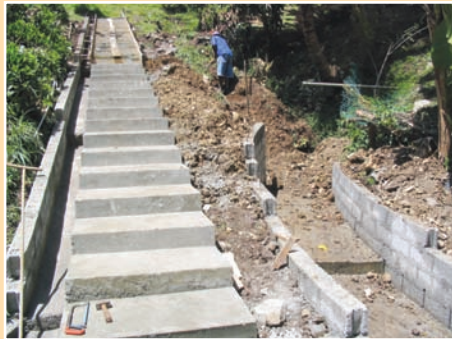
FIGURE 6.19 Examples of footpath and footpath drains being constructed simultaneously
