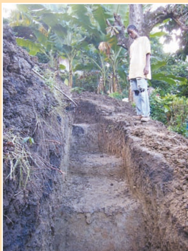
FIGURE 7.18 Self-cleaning stepped drains
