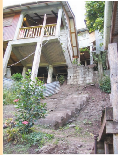
a. Steep slopes can be stable if the depth to bedrock is very shallow.
