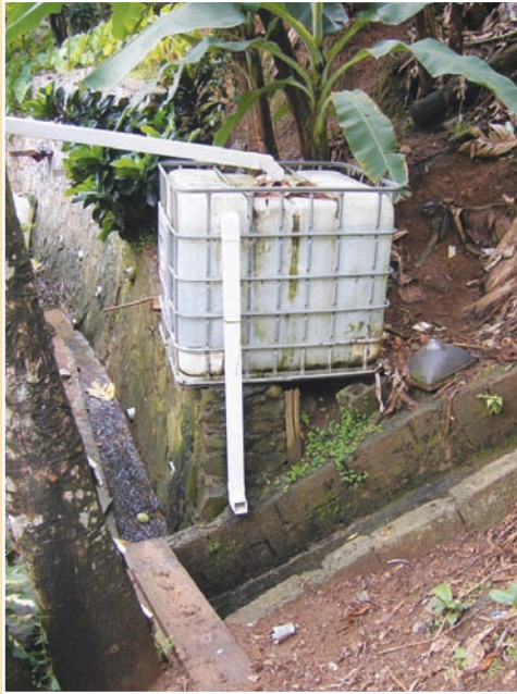
FIGURE 7.26 Connecting water tank overflow pipes to nearby drains
