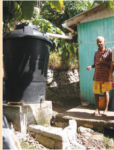
FIGURE 7.26 Connecting water tank overflow pipes to nearby drains
