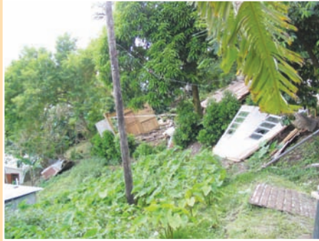
FIGURE 9.9 Convergence of water upslope results in slope instability and property destruction on shallow slope
