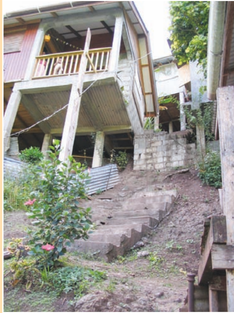
a. Additional loading of a 55-degree slope with an already high housing density increases landslide risk.
