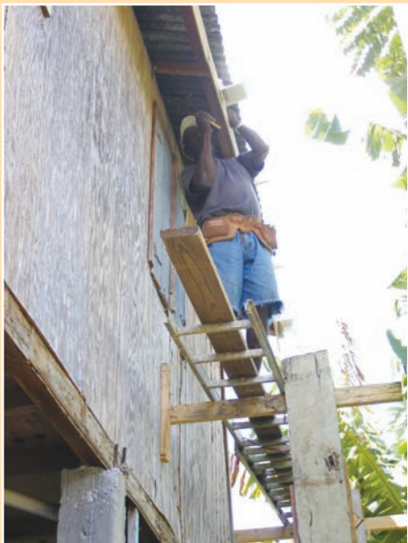
FIGURE 7.3 Modifications to roof structure for roof guttering installation
