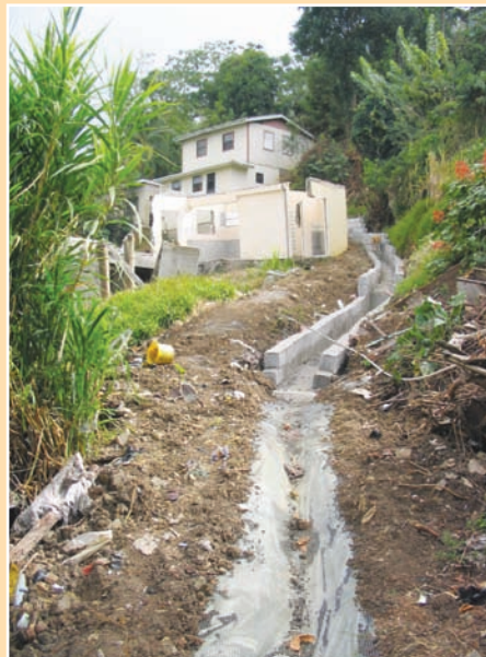
FIGURE 6.31 Combination of block drain and low-cost drain
