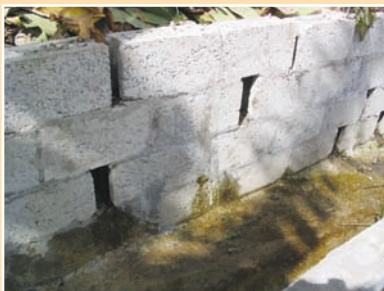
FIGURE 7.20 Weep hole formation
