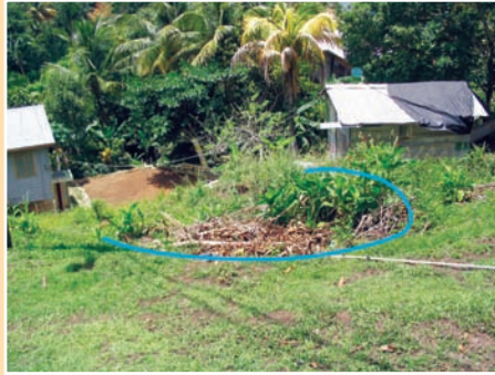
FIGURE 3.23 Shallow rotational slip on an 18-degree slope at the foot of an extensive hillside
