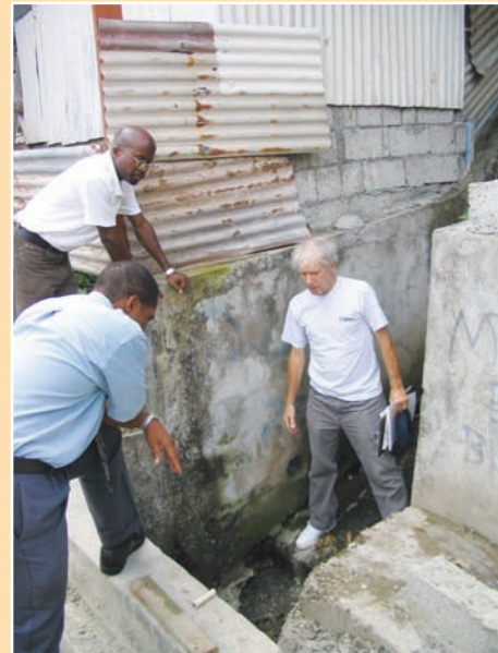
FIGURE 7.38 Choosing a debris trap location
