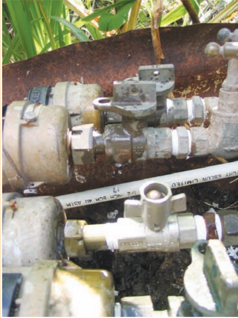
a. Water meters allow an estimation of the volume supplied to the community.
