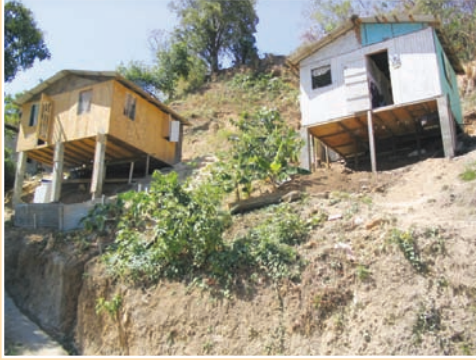
a. Unauthorized housing built on a preexisting landslide within one year of the failure having taken place.
