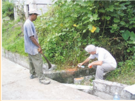
FIGURE 7.14 Clear markings help remove issues of ambiguity for site supervisor
