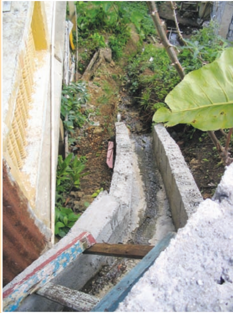
a. Poor design: a newly constructed drain has no planned outflow discharge management. The discharge can serve to increase landslide risk.
