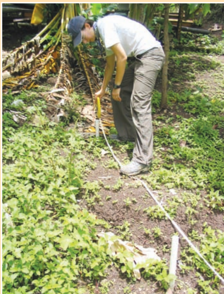
c. Setting out piezometer array.
