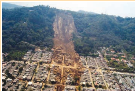
FIGURE 3.6 Aerial view of earthquake-triggered landslide in Las Colinas, El Salvador, January 13, 2001
