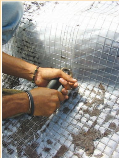
d. Tying mesh lengths with galvanized wire.
