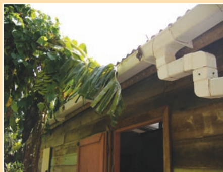
FIGURE 7.4 Downpipe installation detail
