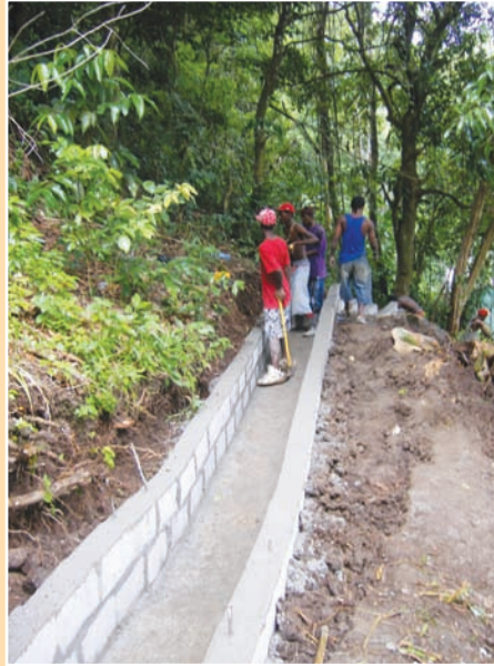
FIGURE 6.17 Main cross-slope intercept drain constructed on a 35 degree slope angle
