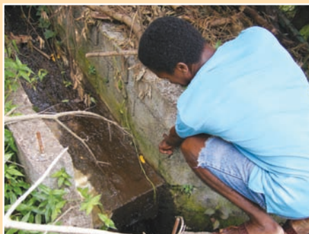
b. Resident indicates maximum flow depth reached during a previous day’s storm.
