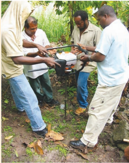
a. Drilling for a piezometer installation.
