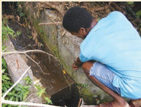
c. Residents can help postproject impact assessment by indicating maximum observed water levels in completed drains after heavy rainfall.
