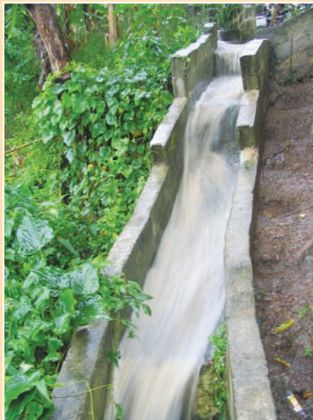
a. Main downslope drain conveys flow from an intercept drain.
