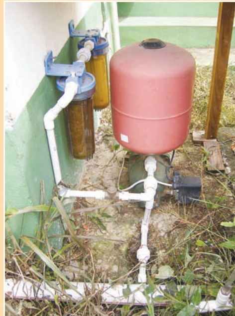
FIGURE 6.36 A system for filtering and purifying water for human consumption
