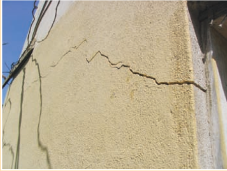
a. Cracks in structure attributable to poor construction (insufficient pile depth).
