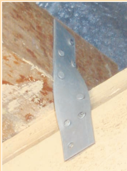
FIGURE 6.44 Roof hurricane strap
