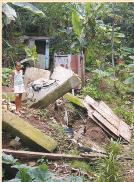
b. Minor landslide where the impact of the debris has destroyed a wooden home.
