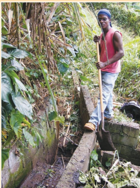
FIGURE 6.22 Postconstruction maintenance: Keeping drains free of debris
