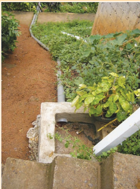
FIGURE 6.41 Concrete chambers connecting water from multiple houses to a single collection point with an outflow pipe to a main drain
