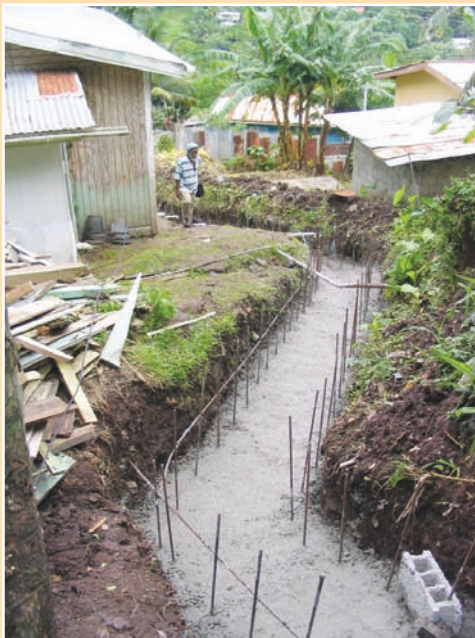
FIGURE 7.27 Examples of drain bases
