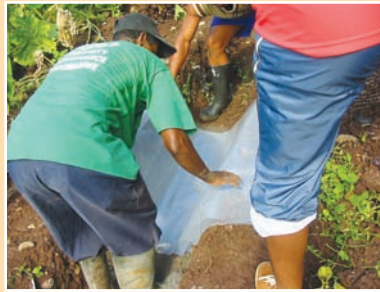
b. Laying plastic lining on sand blinded base.
