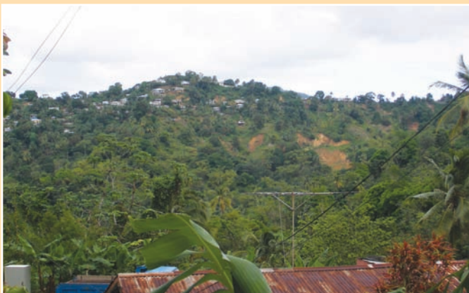
c. Hillside-wide translational landslides St. Lucia triggered by Hurricane Tomas.
