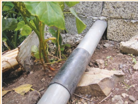
FIGURE 7.29 Using sleeving to join drainage pipe sections
