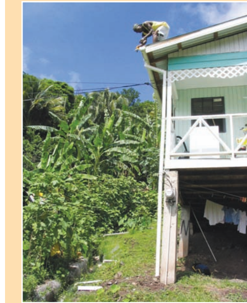
FIGURE 6.34 Retrofitting roof guttering
