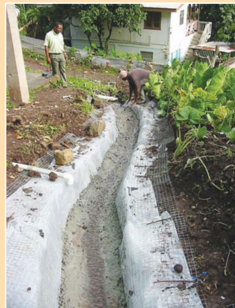
b. Completed drain, with household gray water connections.
