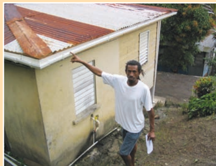
FIGURE 7.23 Newly installed roof guttering
