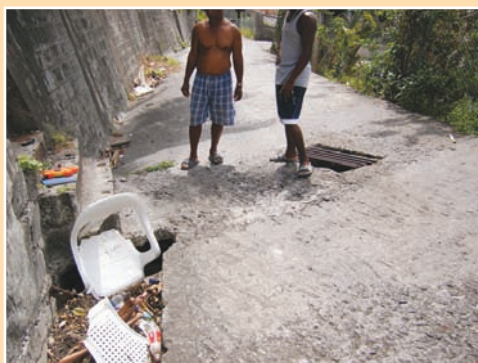
FIGURE 8.18 Debris traps should be installed and cleared regularly
