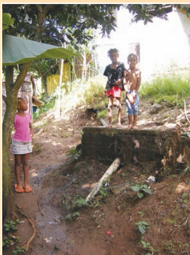
g. Household septic tank discharging directly into the slope.
