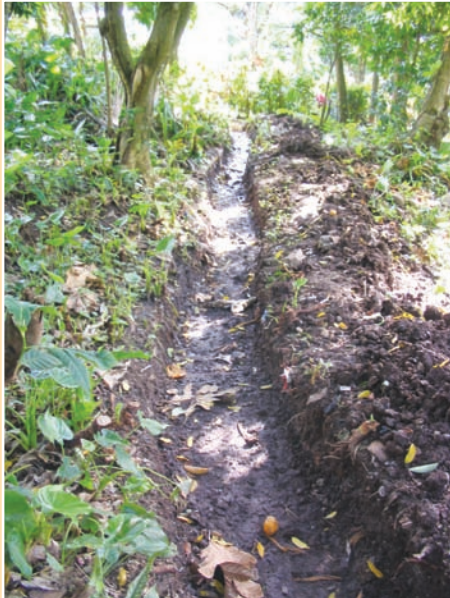
FIGURE 6.30 Community innovation and skills at work after project completion
