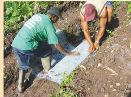
a. Low-cost drain being installed by residents.
