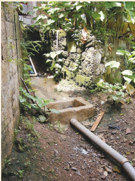
FIGURE 7.25 Concrete connection chambers
