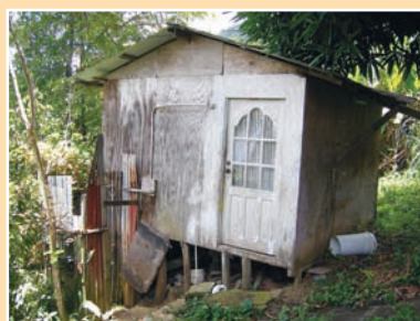
b. Housing stock typical of vulnerable communities.
