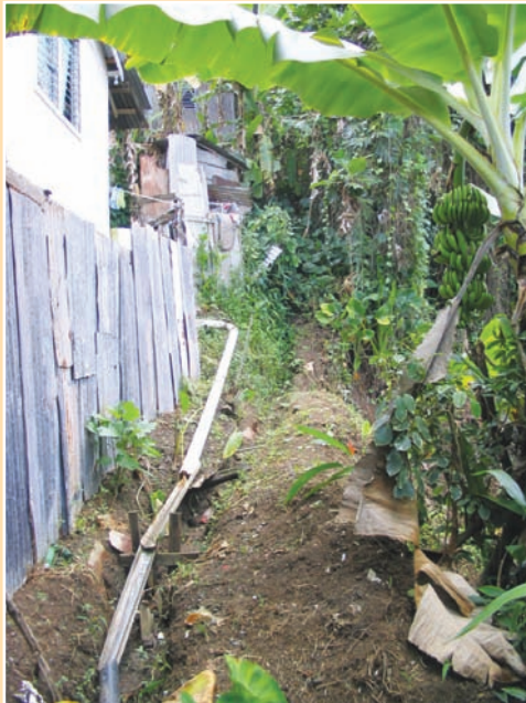
c. It is important to tidy up residents' makeshift gray water connections when drains have been built.
