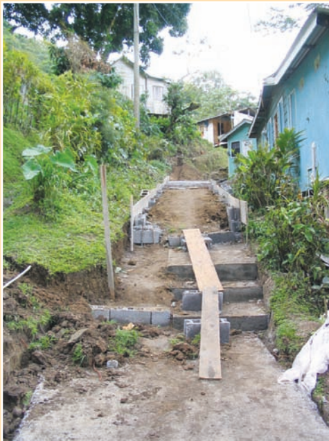
FIGURE 7.28 Providing adequate temporary access to houses during construction
