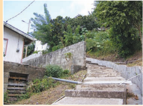
b. Provision should be made for household water connections before a footpath is constructed.
