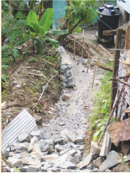
FIGURE 6.26 Rubble wall as part of drain construction
