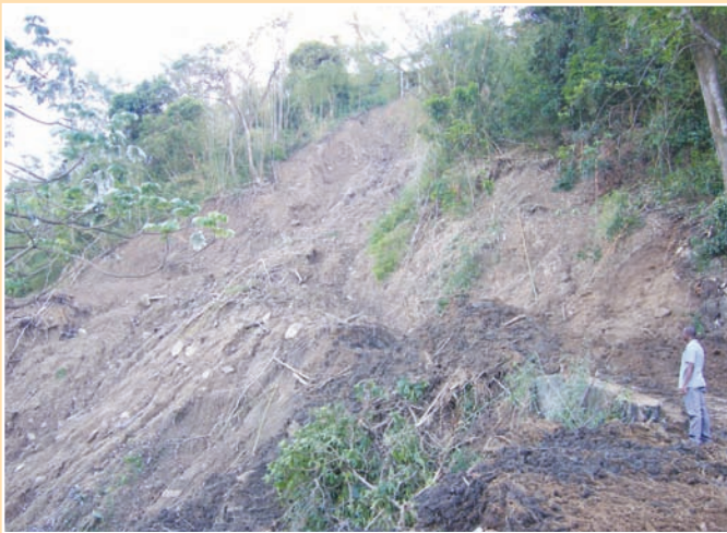
b. Translational slide in St. Lucia triggered by ~500 mm of rainfall in 24 hours associated with Hurricane Tomas (2010); slide caused the loss of a road (center) and significantly damaged houses at the landslide crest.
