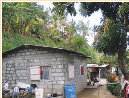
Dense vegetation above the benched slope and a major failure below the property can make it more difficult to estimate the hillslope segment slope angles.
