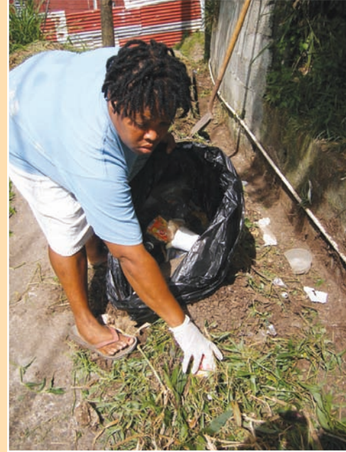
b. Removing vegetation that may block the drain.
