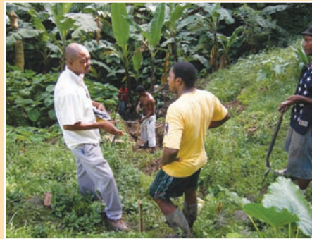
FIGURE 7.15 Site supervisor is critical to project success and to ensuring good construction practice
