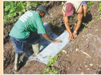
c. Overlaying with galvanized mesh.
