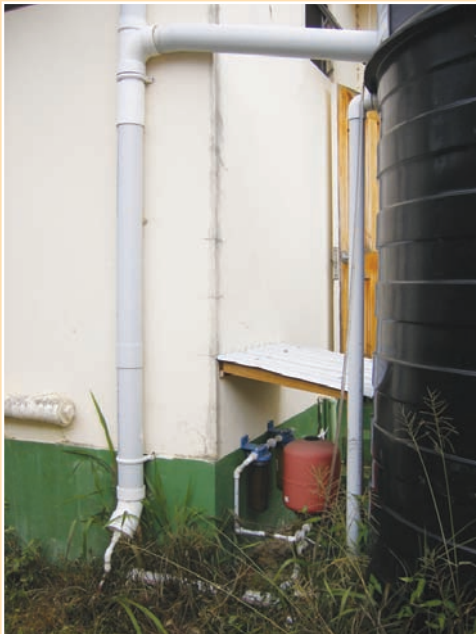
FIGURE 6.36 A system for filtering and purifying water for human consumption
