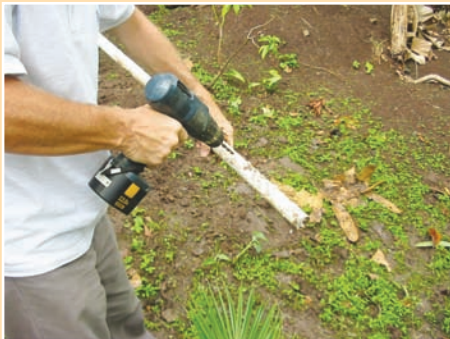
b. Drilling holes in piezometer tube.
