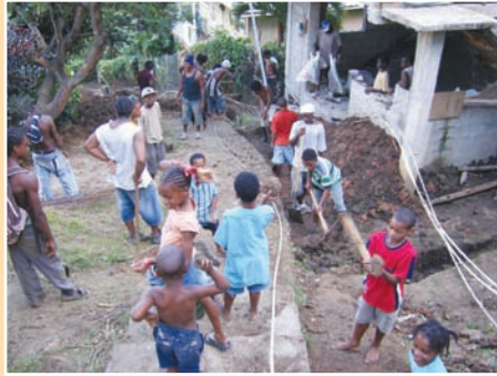
FIGURE 7.16 Supervision issue: Large numbers of residents engaging with contractors
