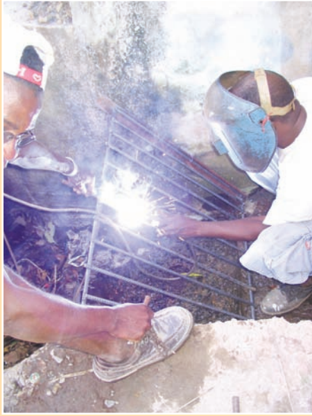
FIGURE 7.39 Welding in-situ and completion of debris trap
