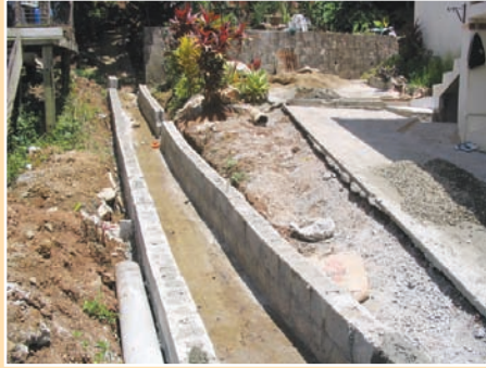
FIGURE 7.19 Finished drain wall height same as adjoining ground surface
