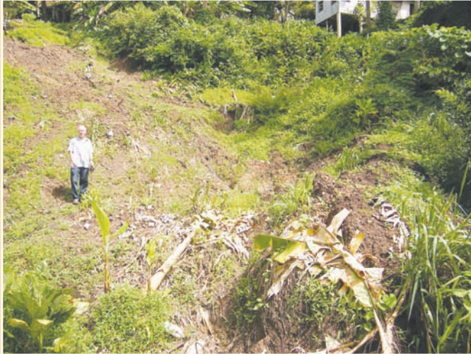
a. Rotational slide in St. Lucia triggered by rainfall during Hurricane Dean (2007) caused the loss of three houses.
