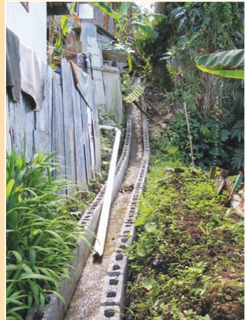
c. It is important to tidy up residents' makeshift gray water connections when drains have been built.
