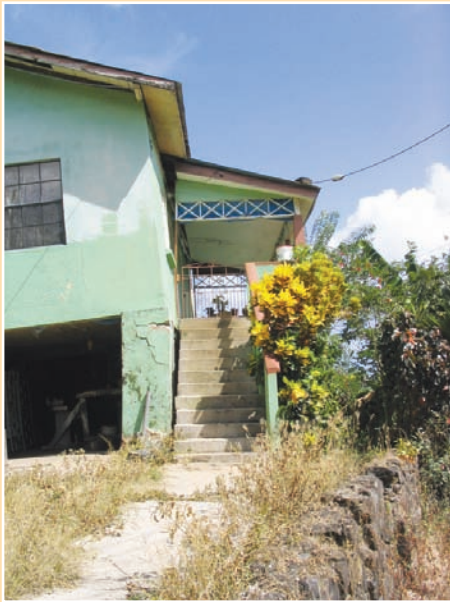
a. Cracks in structure attributable to poor construction (insufficient pile depth).
