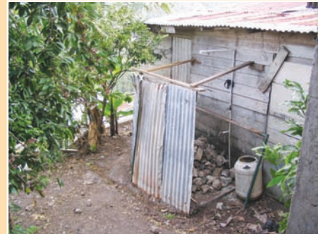
FIGURE 6.38 Capturing gray water from showers and washing machines
