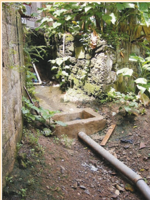
FIGURE 6.41 Concrete chambers connecting water from multiple houses to a single collection point with an outflow pipe to a main drain
