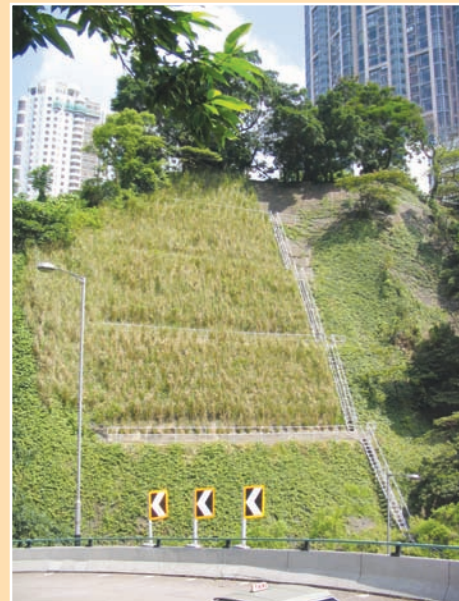
FIGURE 7.37 Bioengineered slope in Hong Kong SAR, China
