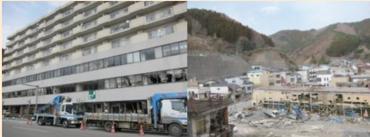
FIGURE 5: Designated evacuation building (left) and evacuation road (right) in Kamaishi
