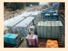
In Rikuzentakata City in Iwate Prefecture, the wastewater treatment plant was severely damaged by the tsunami. But within its service area 400 houses located on higher ground had survived the tsunami. When water supply services resumed, the sewage generated by these 400 houses had nowhere to go. Following a proposal by a private company, the city decided to introduce a movable membrane bioreactor unit, which was quickly installed and began operating within a month.
