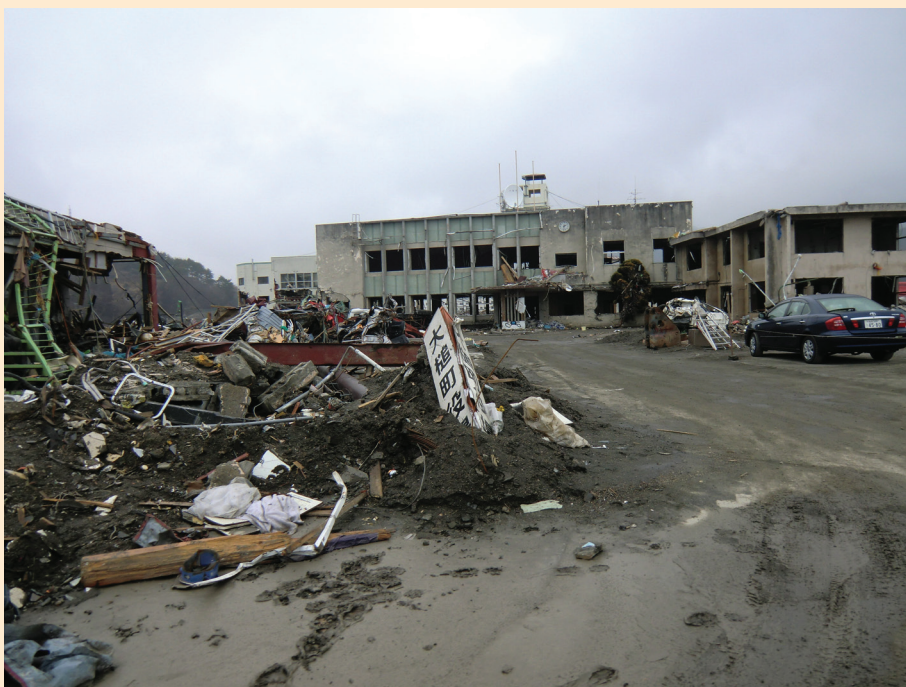
FIGURE 1: The municipal office in Otsuchi City was damaged by the tsunami
