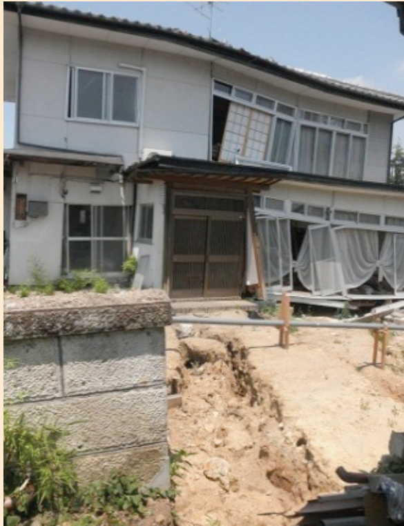
FIGURE 10: Houses damaged by landslides
