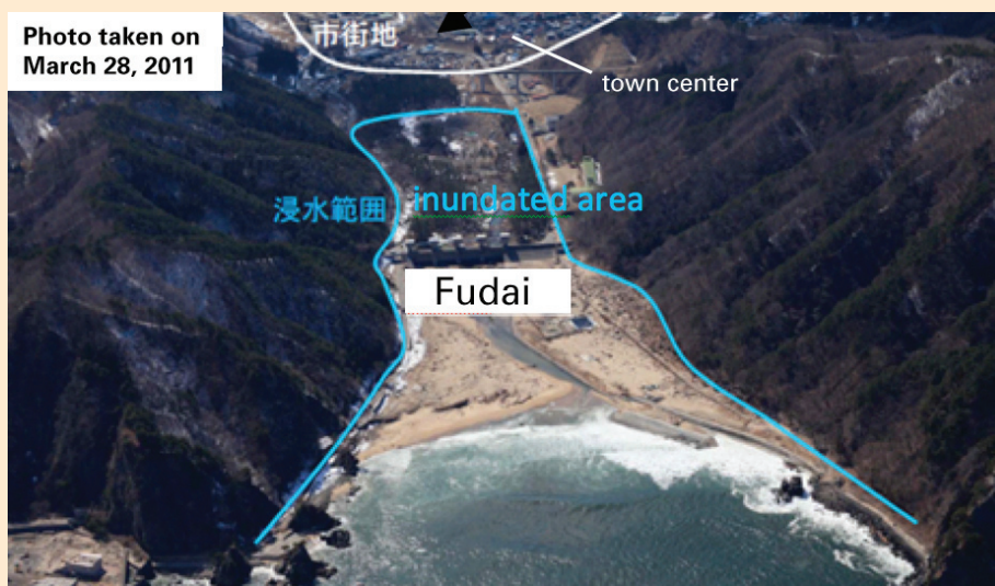
FIGURE 2: Inundation area in Fudai Village, Iwate
