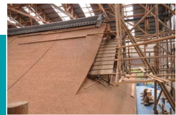
Regular roof retrofitting using traditional techniques and materials
