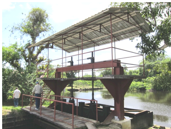
Lama Sluice Rehabilitated under the CAP
