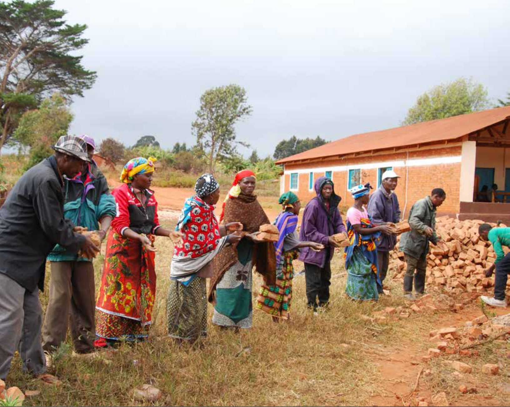
Village of Pomerini, Tanzania— unidentified group recovers red clay bricks still usable from a collapsed house in the village. Photo credit: © Francovlpatto | Dreamstime.com
