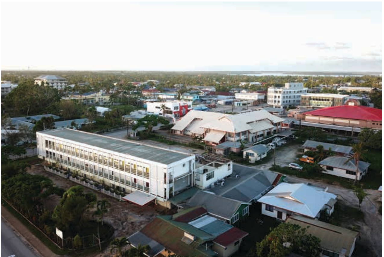
Photo: Malani Wolfgramm/World Bank. Damage to MOET Building, Nuku'alofa.
