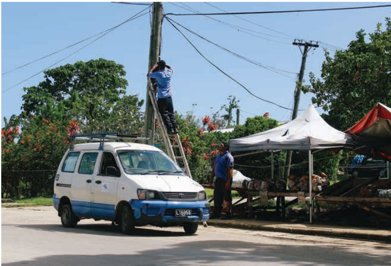
Photo: Malani Wolfgramm/World Bank. Repairing damaged power lines, Tongatapu.
