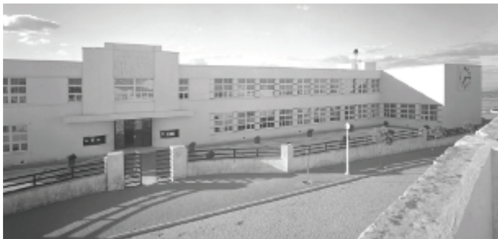
Figure 16: Example of school made of load bearing masonry walls with reinforced concrete floors.
