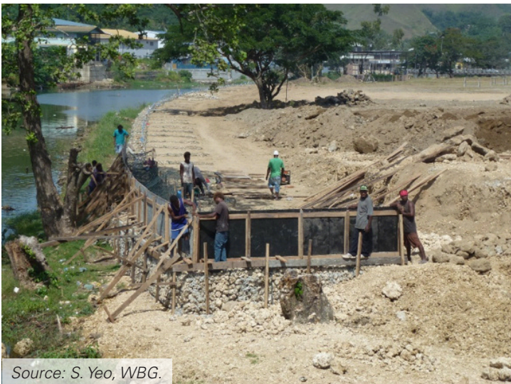
Figure 19. Filling the floodplain and riverbank protection works on one side of the Mataniko River in Honiara
