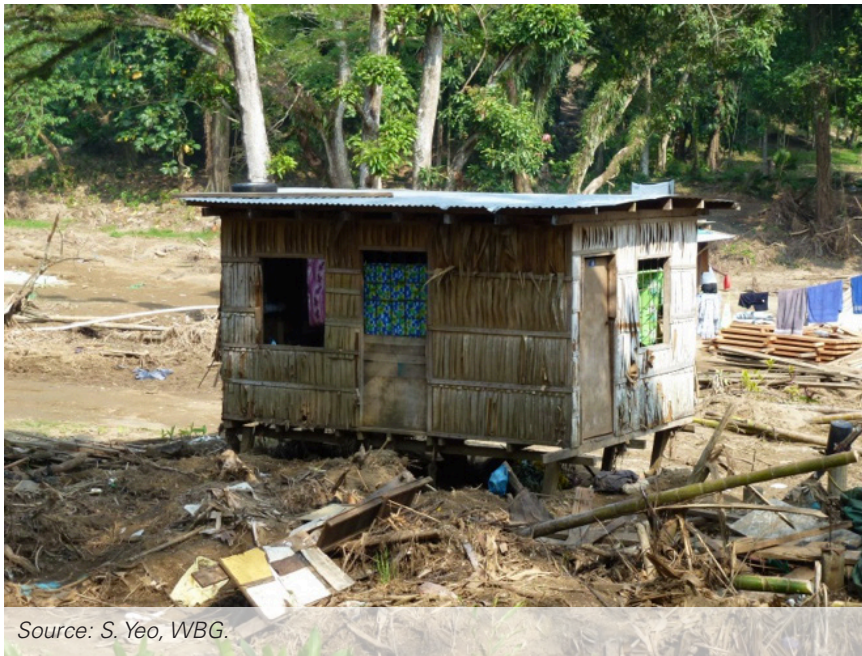
Figure 4. New house on the floodplain, one month after the April 2014 flood, Marble Street, Honiara
