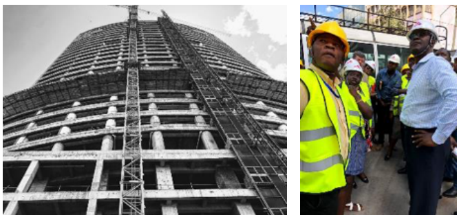
FIGURE 13: Site visit at the new Kenyan Parliament Building in Nairobi
