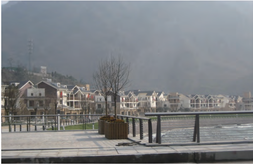
Figure 2.5 Reconstructed Houses in Yingxiu Town Facing the River Source: Authors.
