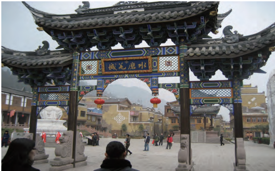
Figure 2.6 The New Look of Shuimo Town after Reconstruction Source: Authors.
