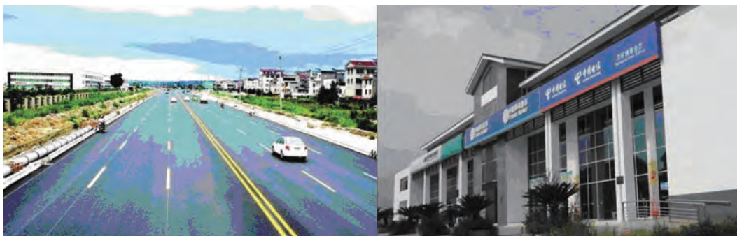
Figure 8.7 Newly Built Beichuan Road (left) and Hanwang Telecommunications Office (right), August 2011
