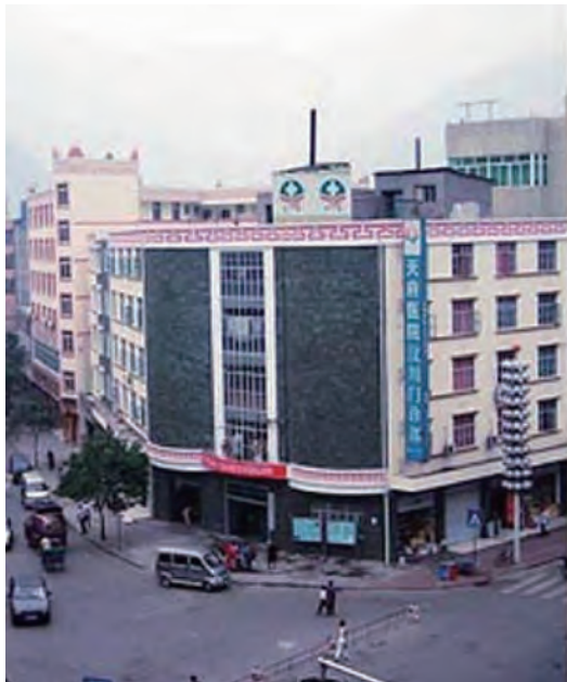
Figure 2.8 Wenchuan Town before the Earthquake
