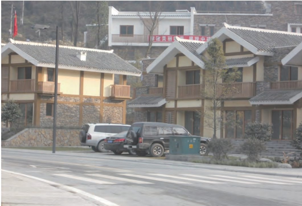
Figure 2.3 Another View of Reconstructed Houses in Yingxiu Town Source: Authors.
