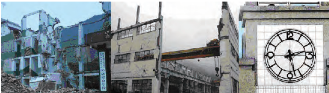
Figure 8.2 Earthquake Damage to Houses and Factories in Hanwang Town
