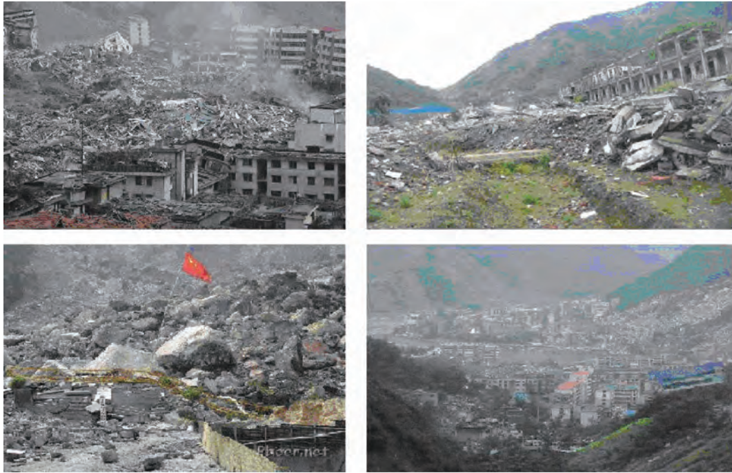
Figure 8.1 Serious Earthquake Damage in Beichuan County
