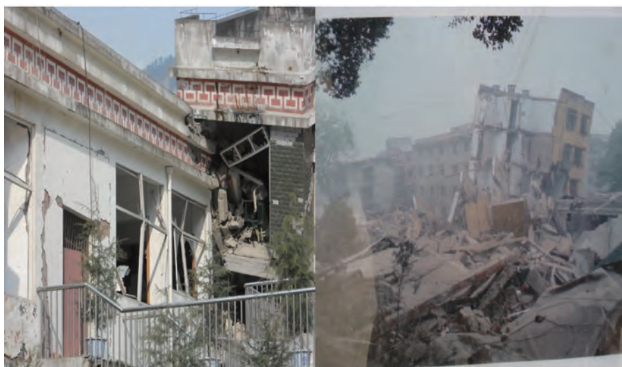
Figure A3.4 Further Views of Wenchuan Earthquake Relics Park
