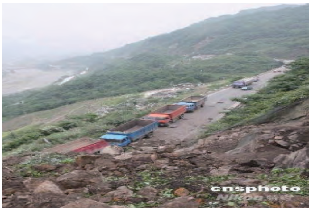
Figure 2.14 Roadway in Wenchuan Disaster Area after the Earthquake Source: http://auto.qq.com/a/20090511/000151_1.htm .
