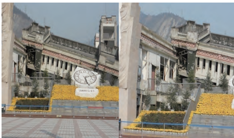
Figure A3.3 Views of Wenchuan Earthquake Relics Park (the original Xuankou Middle School)
