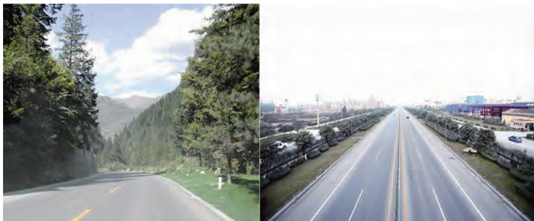
Figure 2.15 Roadways in Wenchuan Disaster Area after Reconstruction Source: http://zhcj.jinmajia.com/article/hyxw/200812/20081200001511.shtml .
