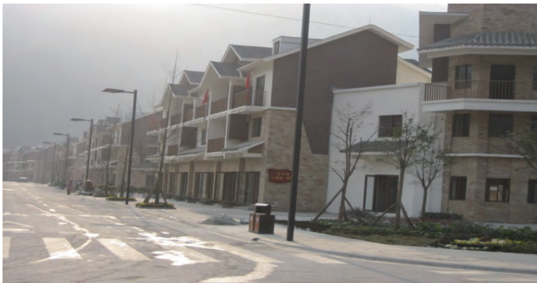
Figure 2.2 Reconstructed Houses in Yingxiu Town Facing Wide New Street
