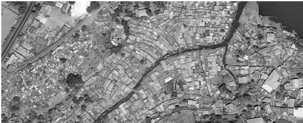
FIGURE 36: Example of High Density Area Near Estuary at Granville Brook/Bomeh Dump Site Prior to Flooding
