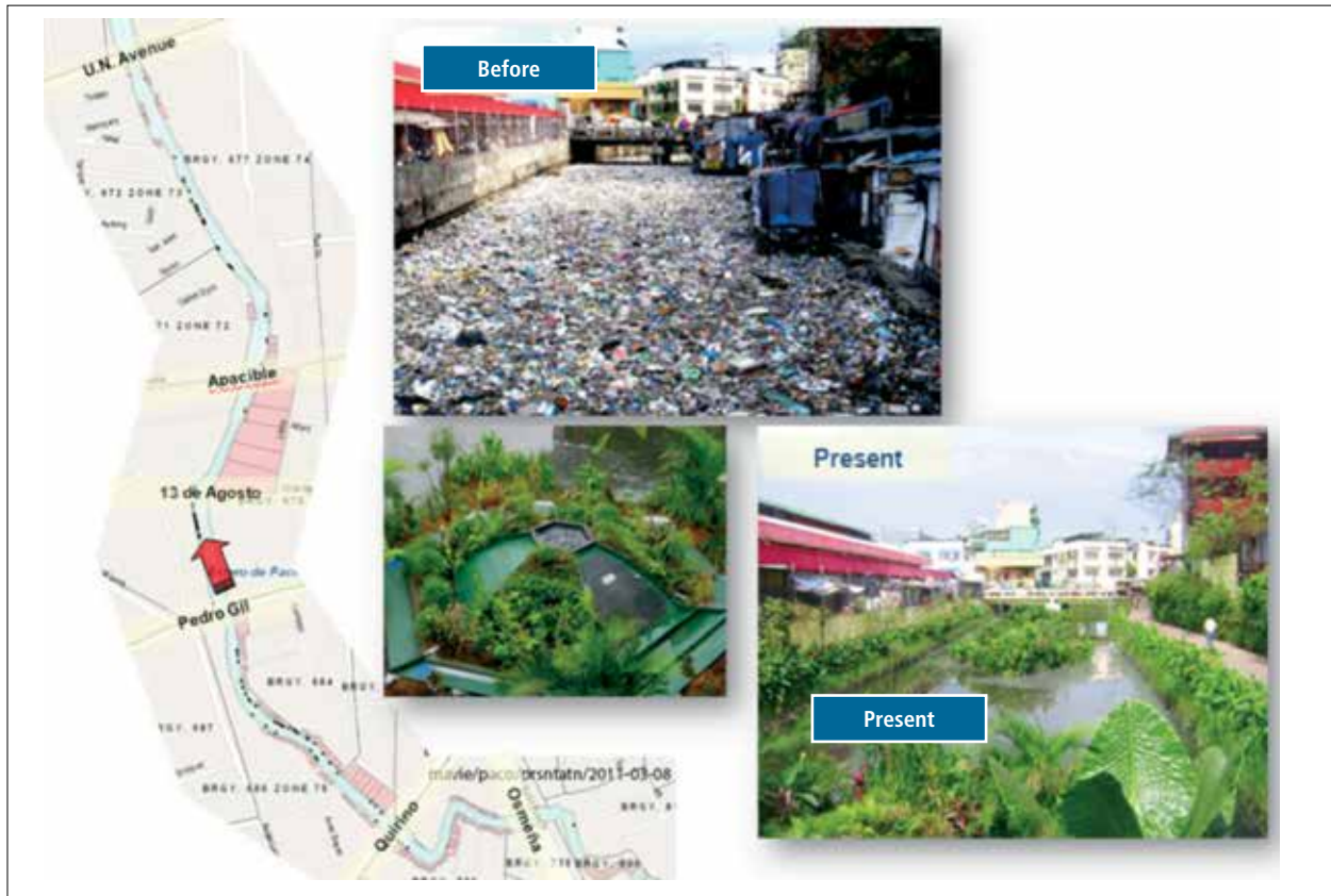
Figure 5 Estero de Paco—Widening, Dredging, and Slope Protection Using Coconets
