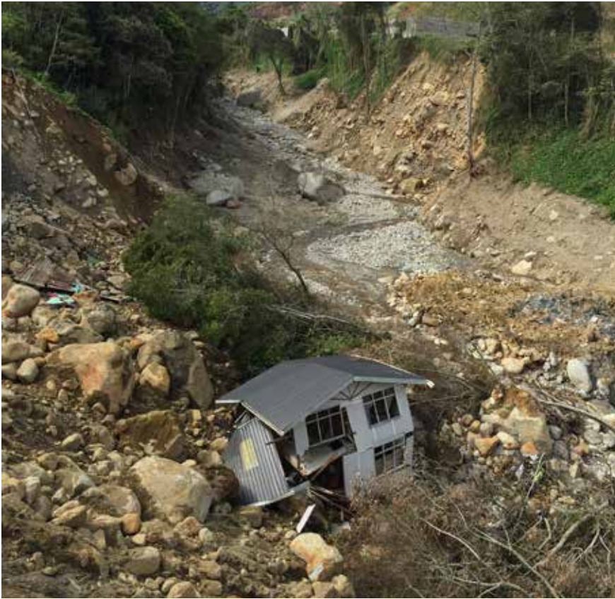
Destroyed house after an earthquake near Mount Kinabalu, Malaysia, July 11, 2015. Photo credit: © Muslianshah Masrie
