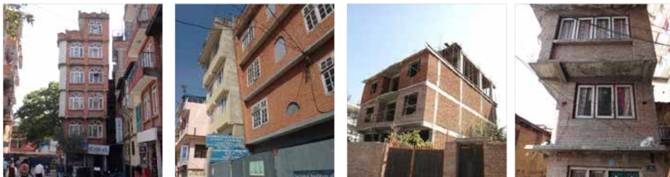
Figure E.3. Buildings in Kathmandu, Nepal, showing typical incrementally expanded building morphologies.
