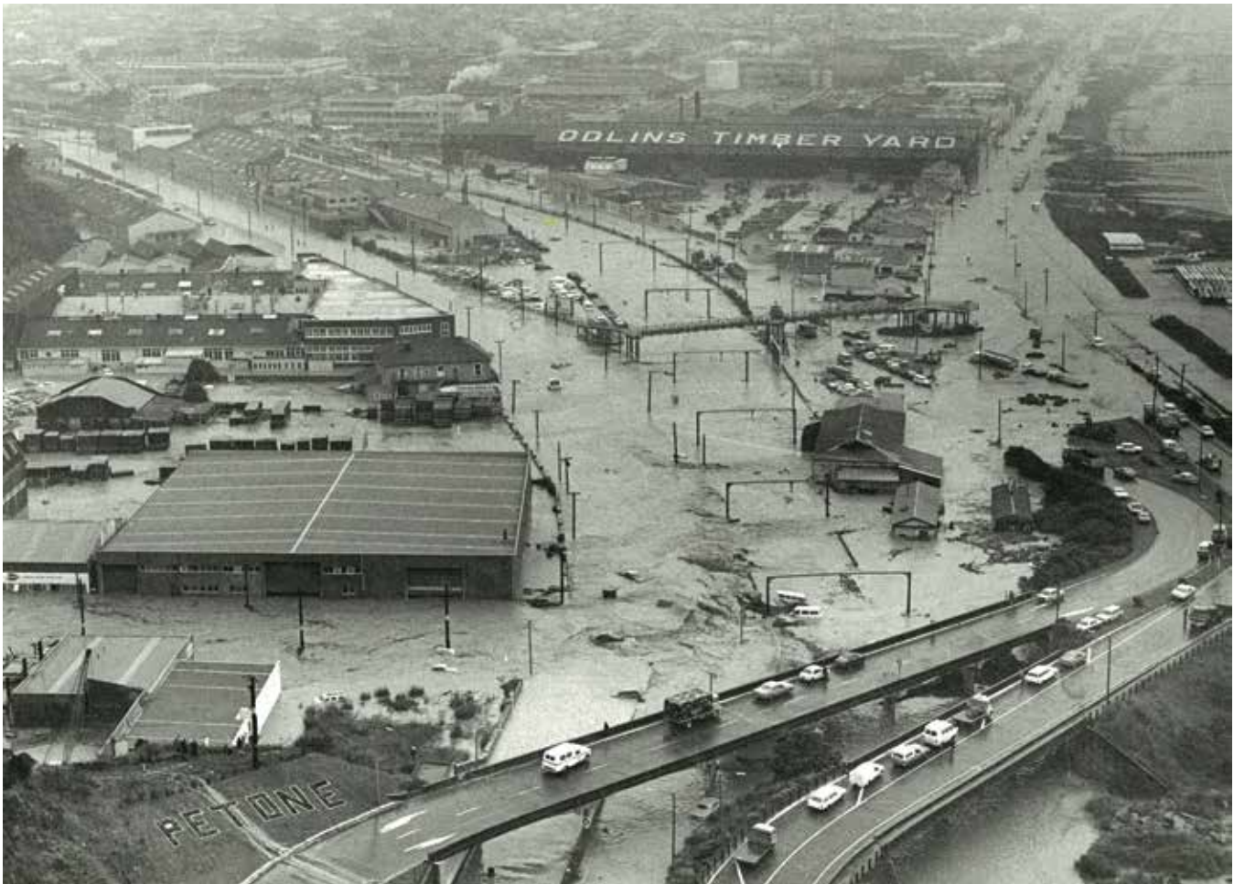
Figure I.5. Flooding from Korokoro Stream in 1976. The Petone Plan Change 29 area extends approximately from the Odlins Timber Yard corner between The Esplanade (located underwater on the far right) and the railway line.
