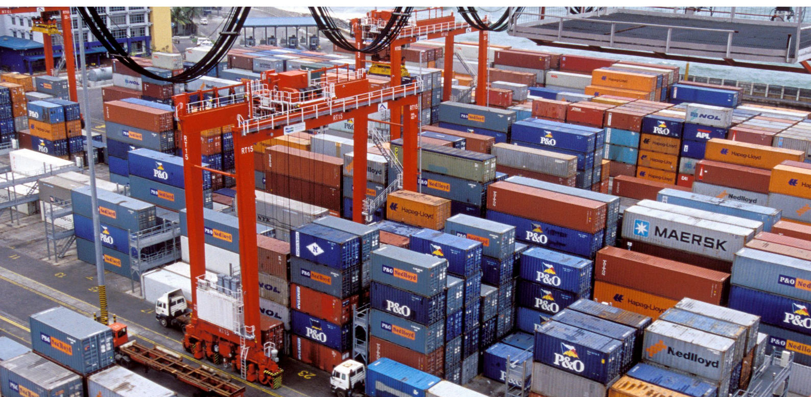
Quay cranes on docks. Sri Lanka. Photo © Dominic Sansoni, World Bank
