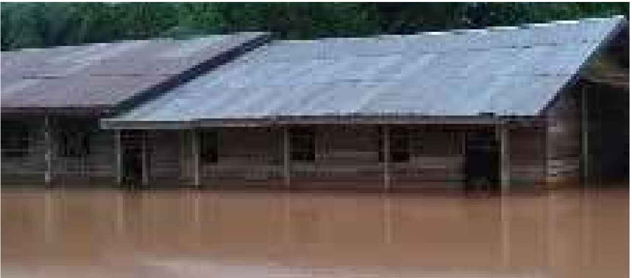
Ban Pong Primary School underwater in Boulapha District, Khammuane Province.
