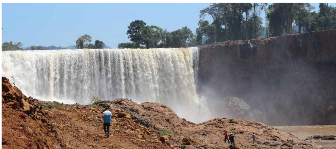
Xe Pong lai Waterfall, showing the damaged area at the base of the waterfall, Sanamxay District, Attapeu Province.
