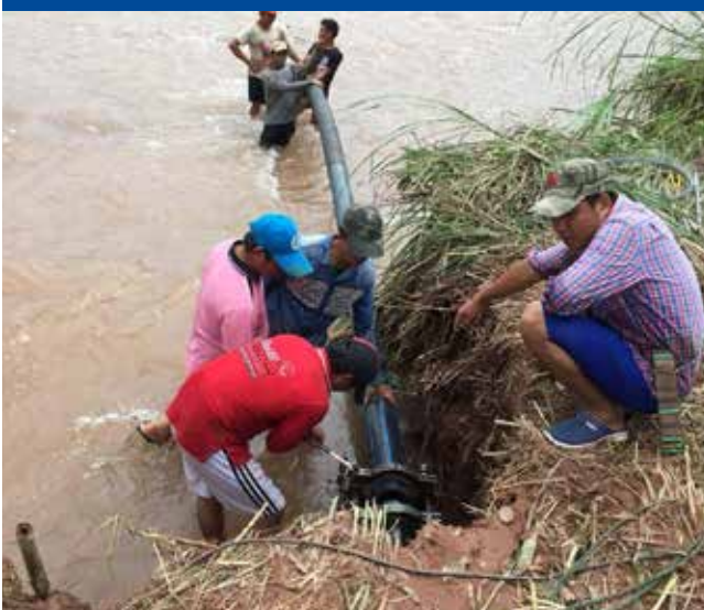
Nam Papa team of Beng District, Oudomxay Province, carries out emergency repairs to damaged urban water supply systems.
